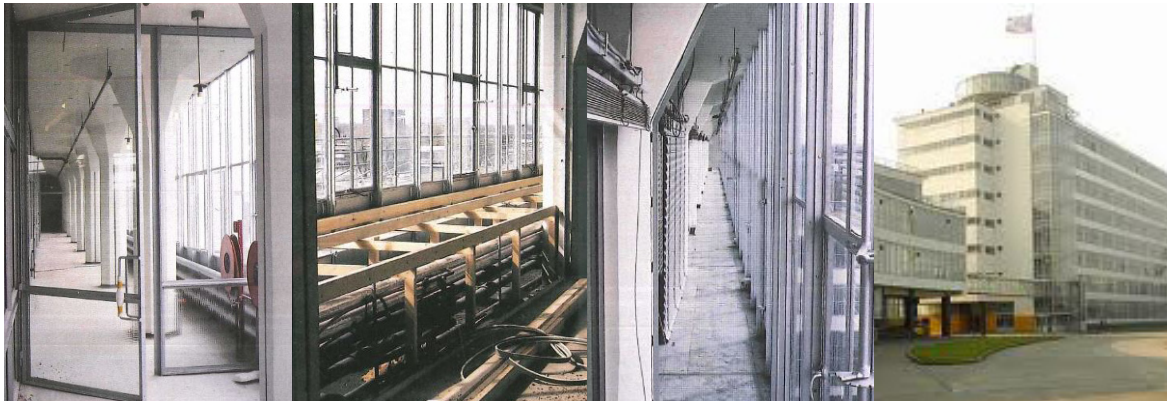
Fig. 23. Van Nelle fabriek, climate facade with ducts under floor (Wilschut, 2001, p. 43).
