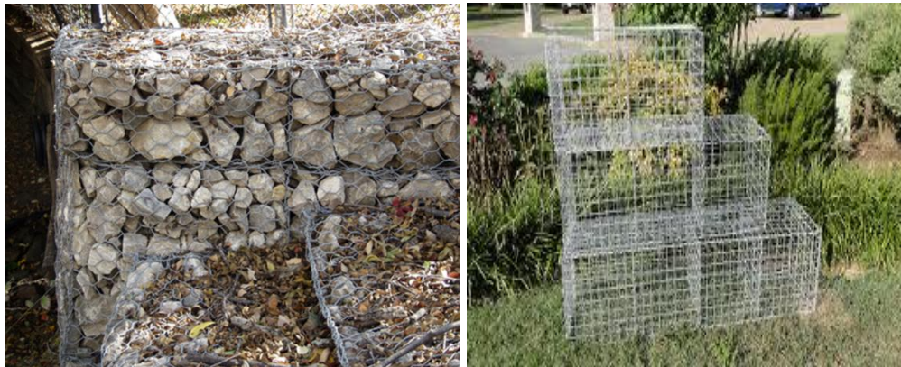
Figure 46. Gabions (left) and gabions meshed cages (right) (DWA, 2013)
