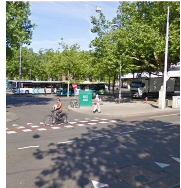
The bus platform before it was covered
