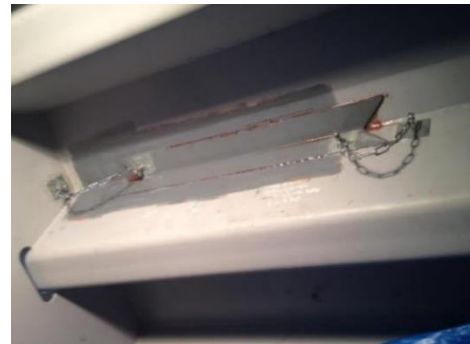
Figure 1.3: Implementation of Cold Repair method using steel on Galecopper bridge [8]
