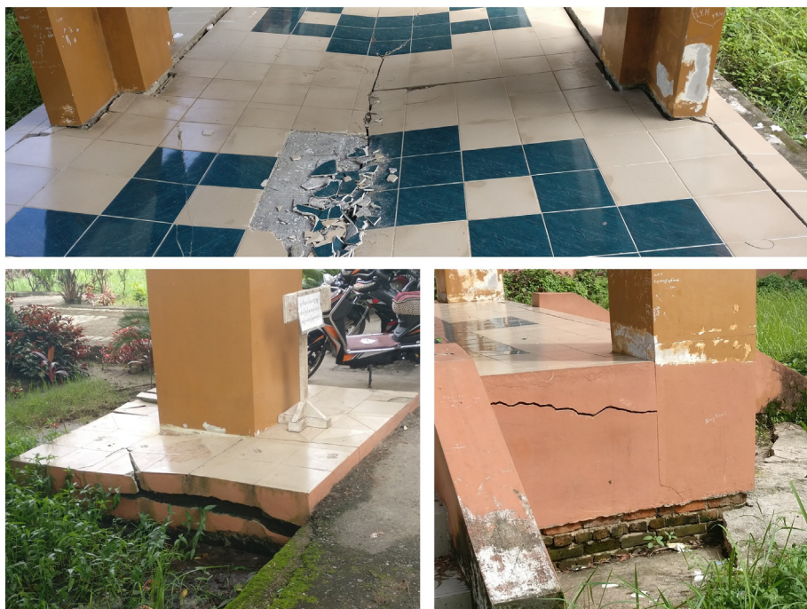
Fig. 8. Damage found at the administration building of Dagon University, likely caused by subsidence originating from layers above the foundation zone of the building. Dagon University is located at the North side of the subsidence zone marked with A. The PS near and over the building indicate subsidence rates near 45 mm/yr, and the building was constructed in 2005.
