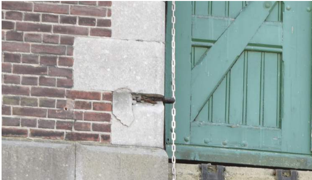
Damage caused by rust in sandstone along the loading door
