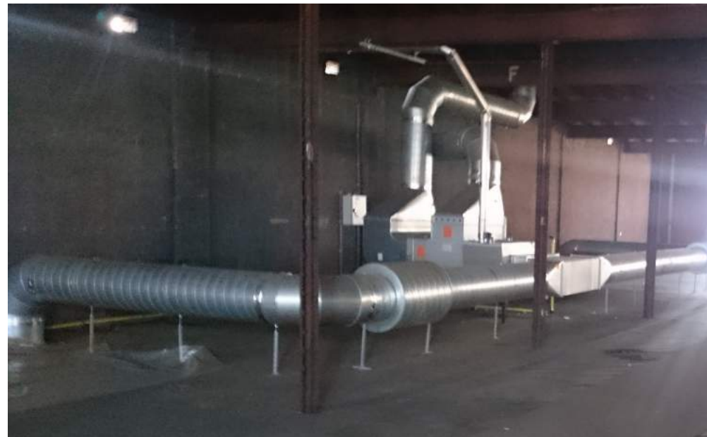
Unit for ventilation and heating
