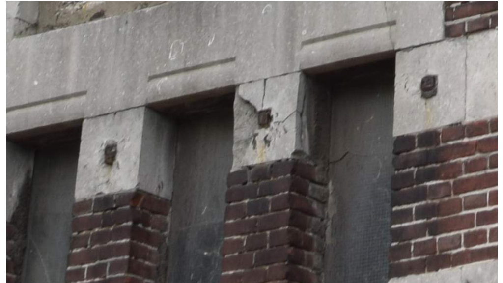
Damage caused by rust in sandstone along the windows
