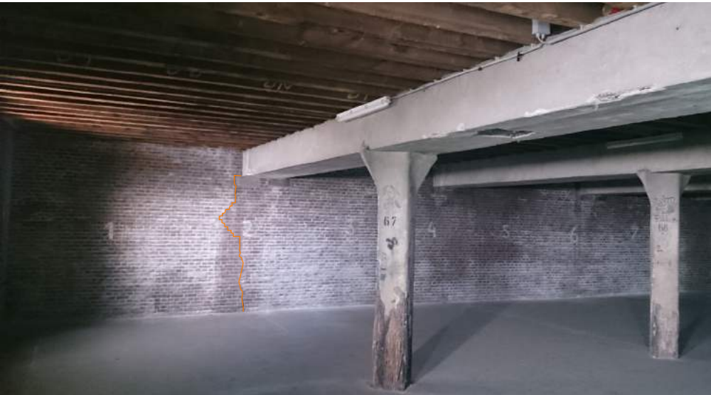
Cracks underneath the beam
