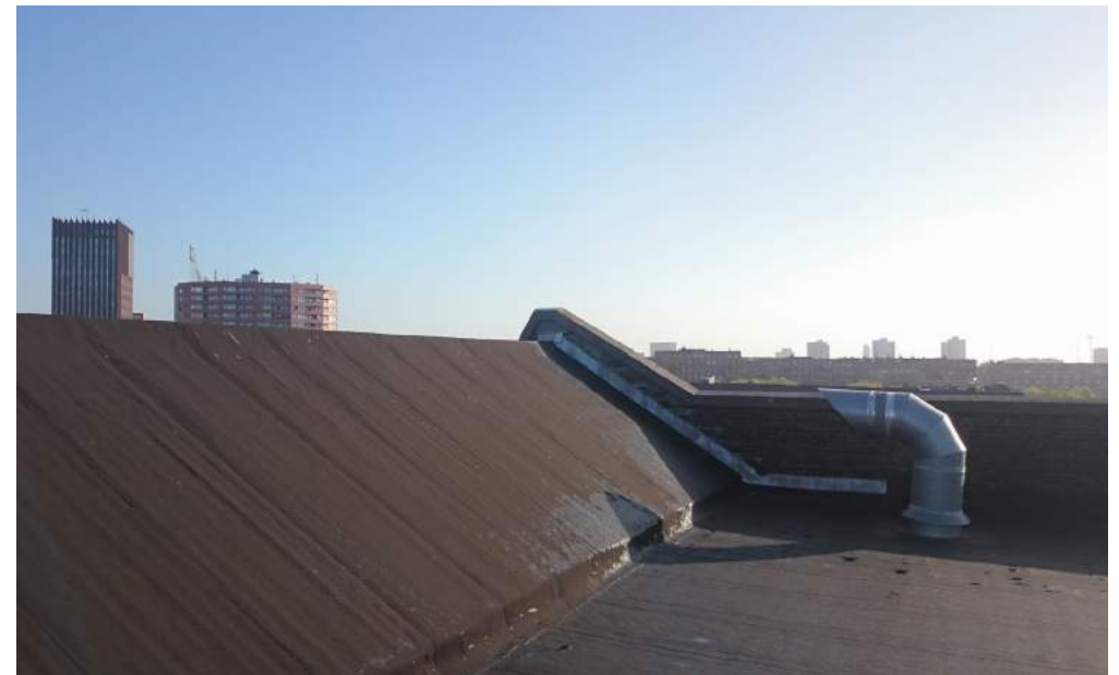
Supply and return ducts on the roof
