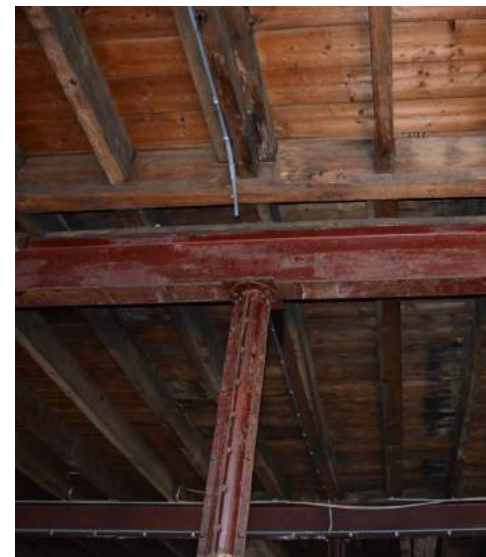
Rust on the main structure of the fifth floor (B. Bronswijk)
