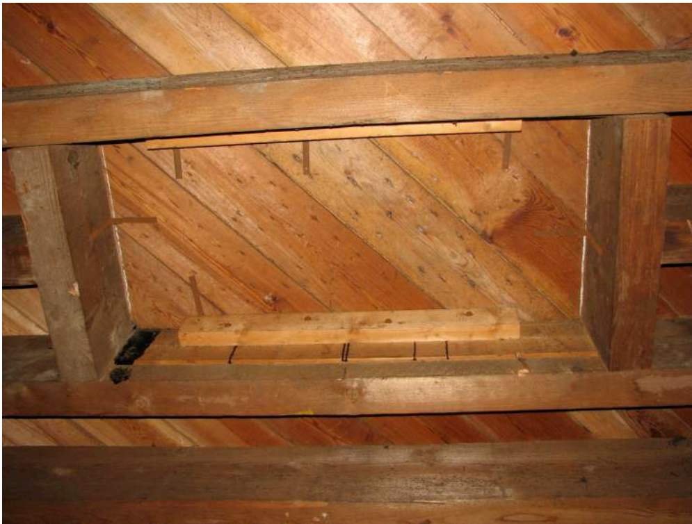
Bottom side of the floor with diagonally boards (S. Fischer)
