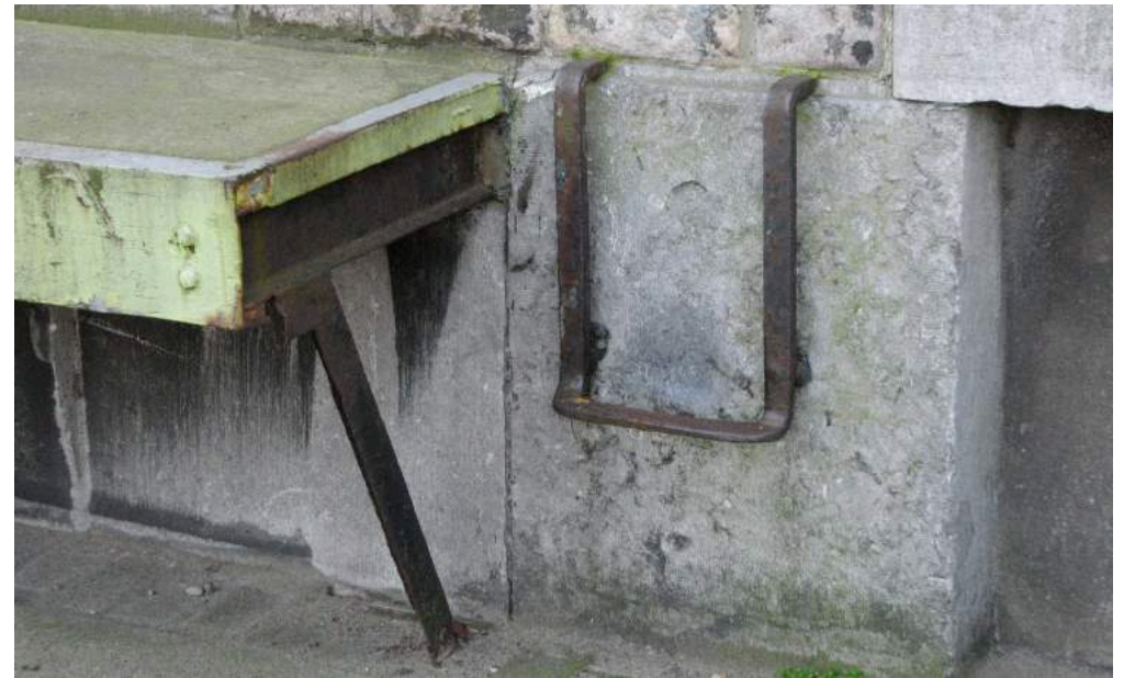
Rust elements of the loading platform and the stair (S. Fischer)
