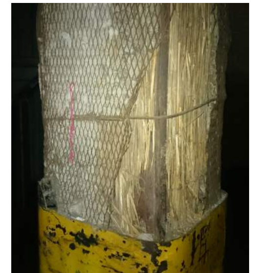
Damage to the fire-resistant cladding
