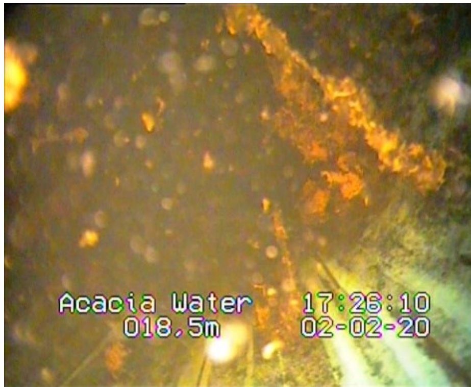
Figure 8.1: Large biofilm depicted near the middle filter screen shot after the first clogging event from infiltration period one.
