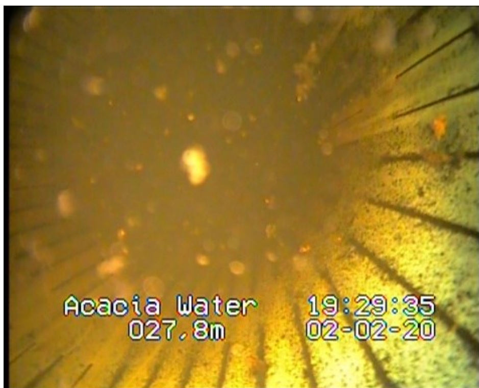
Figure 8.2: Dark material (organic) within filter slots with staining on the well interior.
