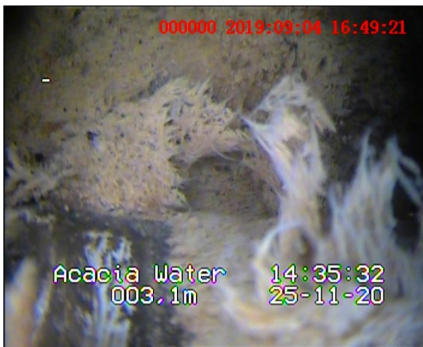
Figure 5.3: Several shots of the conditions within the standpipe taken November 25 th , 2020 after a 41-day standstill. A thick mat of microbial deposits covered the pipe interior and seemed to thicken with depth. The image below shows the standpipe material colour.
