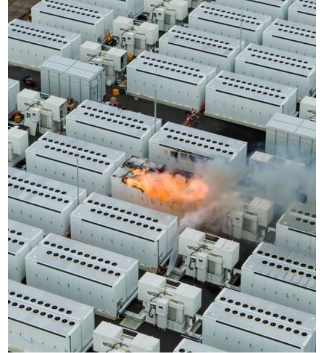
Figure 35. Fire caused by faulty battery. Reprinted from Aroged [17].
