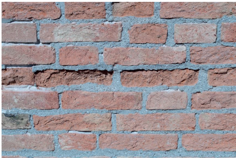
Figure 1.2: Example of damage to brick partly caused by replacement of the pointing with not compatible mortar.
