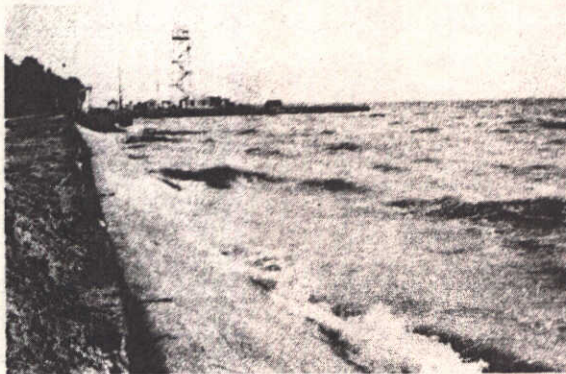
Lok-Gard revetment, Cedarhurst, Md.
