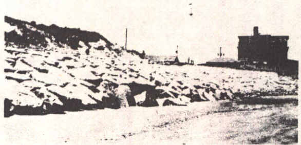
Rock revetment at Chesapeake Bay, Md.
