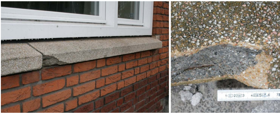
Fig. 6. Typical mass-produced precast concrete windowsill dating from the 1930s. Left: Overview of a windowsill with a broken off corner. Right: Close-up of a damaged windowsill showing a coloured facing layer and a grey backing concrete. Due to soiling, the original colour changed from a beige-orange colour to a more dirty shade of green.
