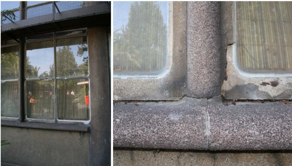
Fig. 5. Precast concrete elements (window frame and sill, plinth, columns etc.) made by Schokbeton N.V., using different ground aggregates to alter the colour of the concrete (Zoo Blijdorp, architect S. van Ravesteyn, 1939). Left: overview façade. Right: beige-sandstone coloured window frame and a more pink-purple coloured windowsill and column. Partially spalling and cracking has occurred, exposing the reinforcement, and discolouration due to soiling.
