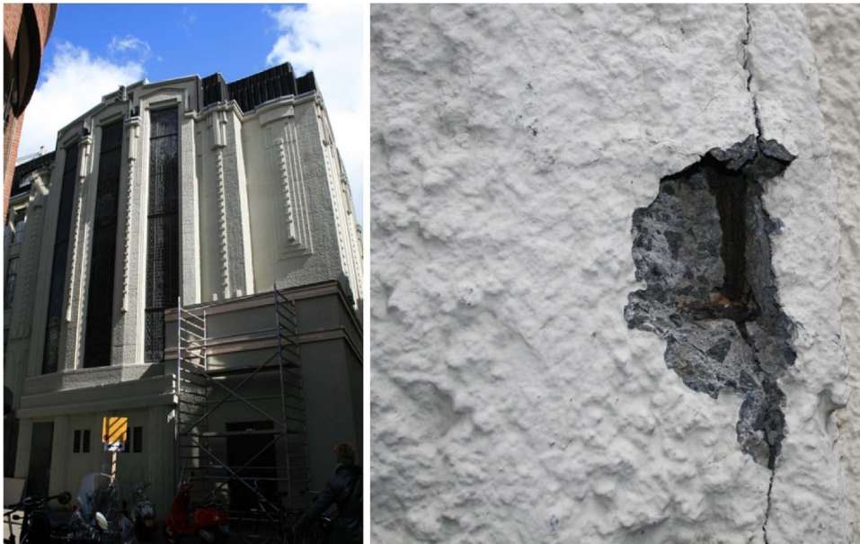
Fig. 4. One of the first Dutch buildings with exposed concrete, yet currently painted (architect A. Moen, 1915). Left: Overview of the rear façade. Right: Detail of a pilaster with spalling, cracking and corrosion, showing the original concrete made with crushed porphyry and with a tooled surface under a layer of paint.
