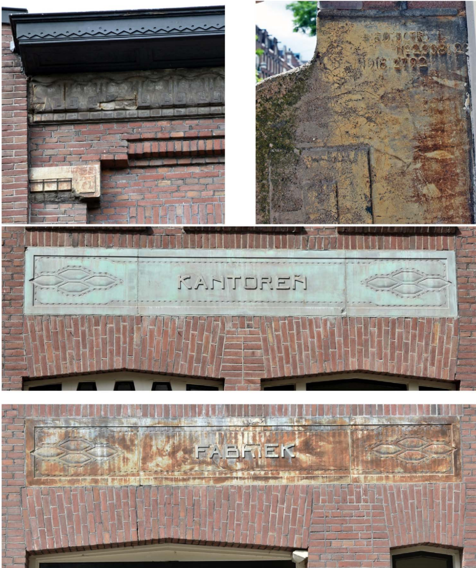
Fig. 3. Overview of precast metallised concrete elements in a former factory (architect C. Tenenti, Amsterdam, 1921). Top left: Cornice made with dark coloured metallised concrete and capital with a sand stone coloured metallised concrete with local darker patches. Top right: detail of a yellow-brown coloured base, with visible inscription of the year and patent number. Middle: Green copper coloured precast metallised concrete sign above entrance for offices. Bottom: Multicolour (green, rust coloured) sign above the entrance to the factory.
