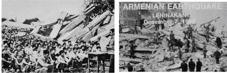
Figure 2-1 Collapse of poorly designed and constructed precast concrete building
