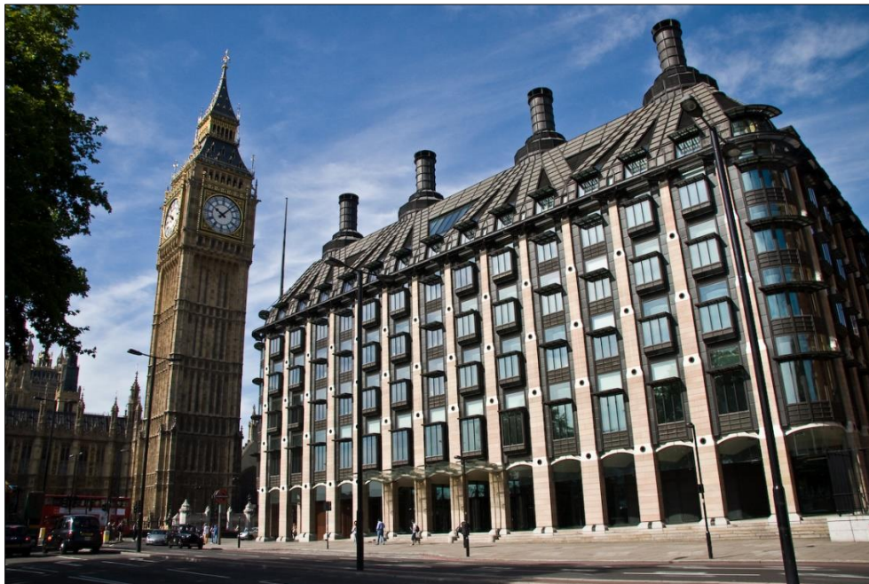
Figure 7: Nickel aluminium bronze window frames, Portcullis House (London) [1].
