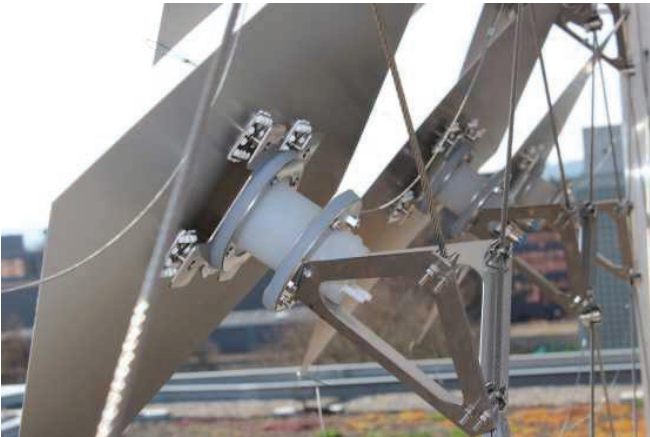
Figure 18: photovoltaic sunshading system embedded with soft robotics
