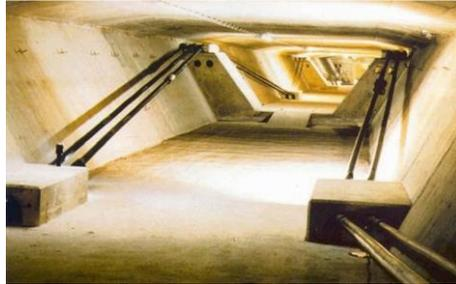
FIGURE 61, PRESTRESSING WIRES IN BOX GIRDER BRIDGE (TENSACCIAI, 2007)
