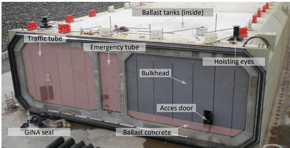
FIGURE 8, TYPICAL IMMERSED TUNNEL ELEMENT (ECPLAZA, 2020)
