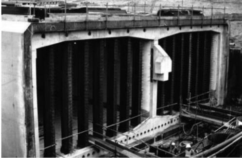
**FIGURE 36, TUNNEL ELEMENT FACE INCLUDING NOSE (BABER & LUNISS, 2013)**
