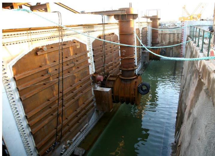
FIGURE 26, ACCESS SHAFT PLACED ON BULKHEAD (TEC, 2017)
