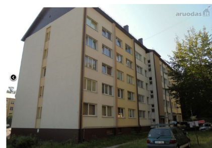
Fig. 2.78. Renovated "Khrushchevka" but adding top floor Source: https://www.aruodas.lt/
