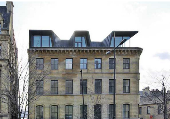
Fig. 3.65. Rooftop extension Source: http://archidesignclub.com/
