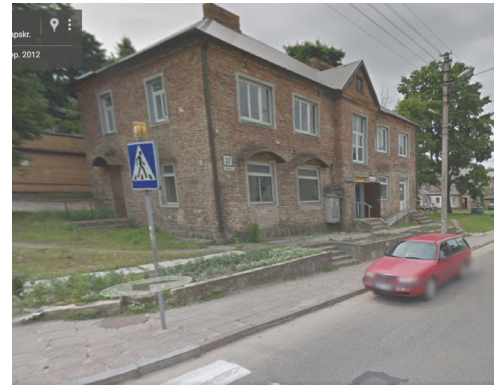
Fig. 3.28. "Stand alone" building Source: Googlemaps street view
