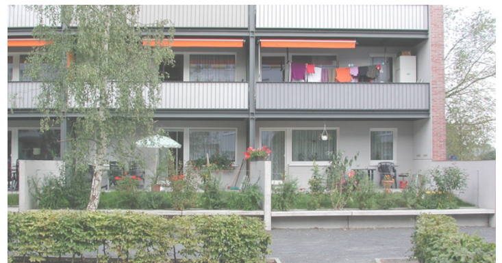
Fig. 3.59 Private gardens/terraces of housing estates in Leinefelde, Germany Source: http://www.muck-petzet.com/
