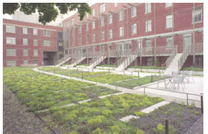
Fig. 3.79. Courtyard of housing block Source: http://www.greenroofs.com/
