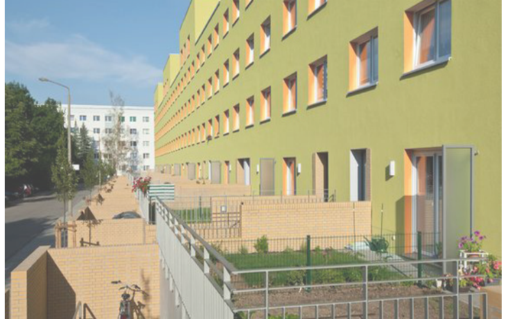
Fig. 3.58. Private entrances of housing estates in Halle, Germany Source: http://www.jeder-qm-du.de/
