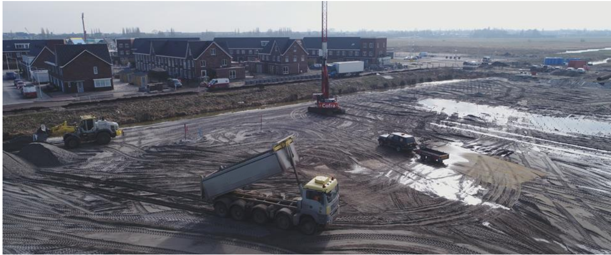
Figure 17: Execution soil improvement (Geonius, 2017)
