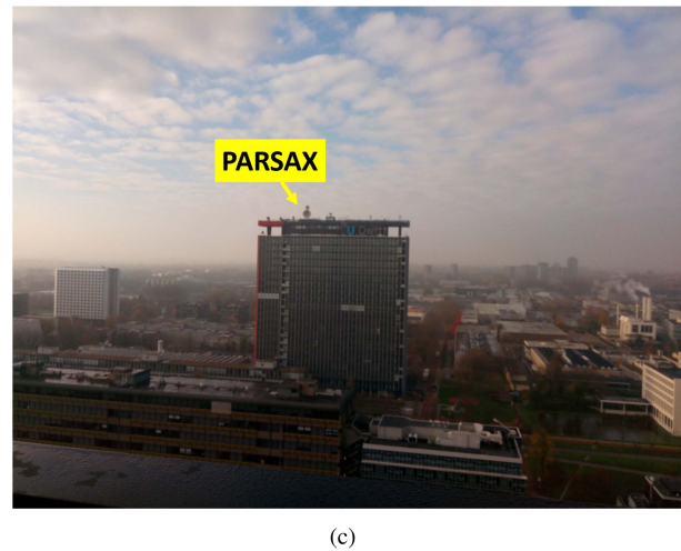
Fig. 11. (a) PARSAX transmit antenna pointed towards the receiver which is shown in (b), and (c) PARSAX as it is seen from the receiver side.
