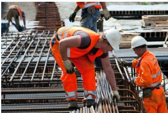
Figure 7: Construction worker (Rodenburg , 2013)
