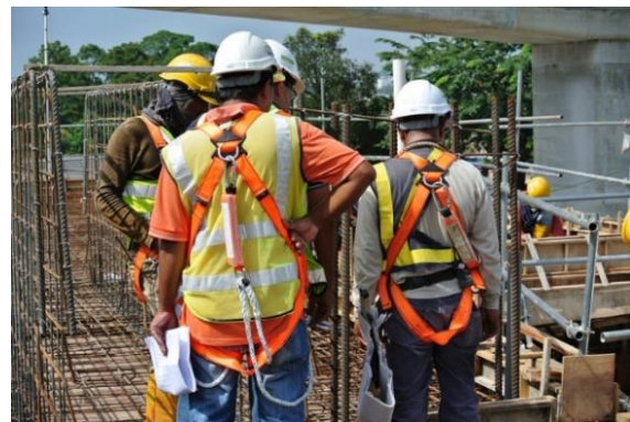
Figure 8: Construction workers with harness (Worldsafety2018, 2019)
