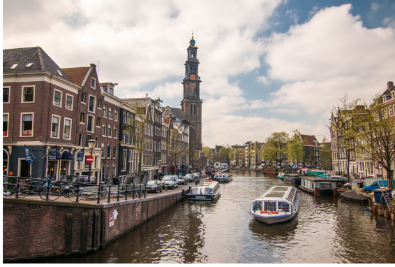
Fig. 1. Quay wall in Amsterdam.
