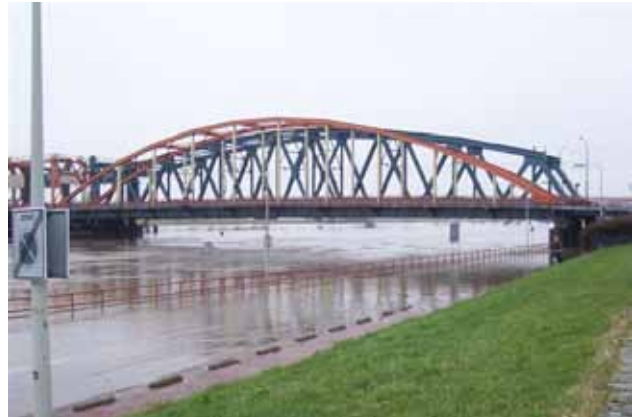
Fig. 2.18: Passageway flooded. (Photo made by author)
