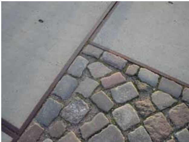
Fig. 3.36: Harbor materialisation of Hafencuty used as reference. (Photo made by author)
