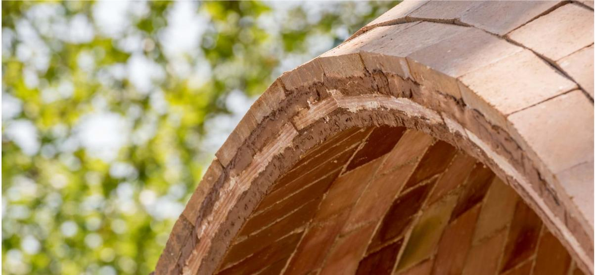
**Figure 1:** Example of thin-tile vaults: Droneport.
