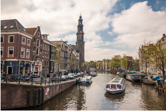
Fig. 1. Quay wall in Amsterdam.
