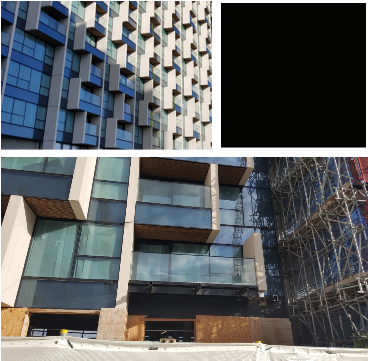
Figure 5.1.15 Building foto's (Scheldebouw, 2019)
