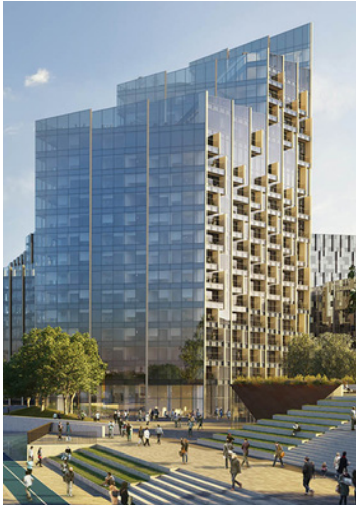
Figure 5.1.16 Building foto's (Scheldebouw, 2019)
