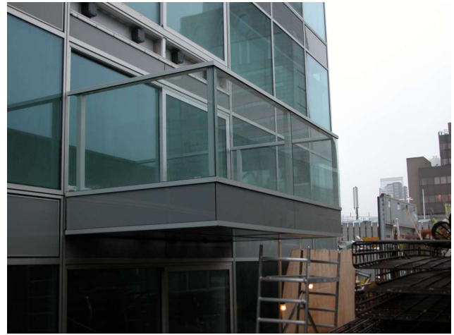
Figure 5.1.09 Building foto's (Scheldebouw, 2019)
