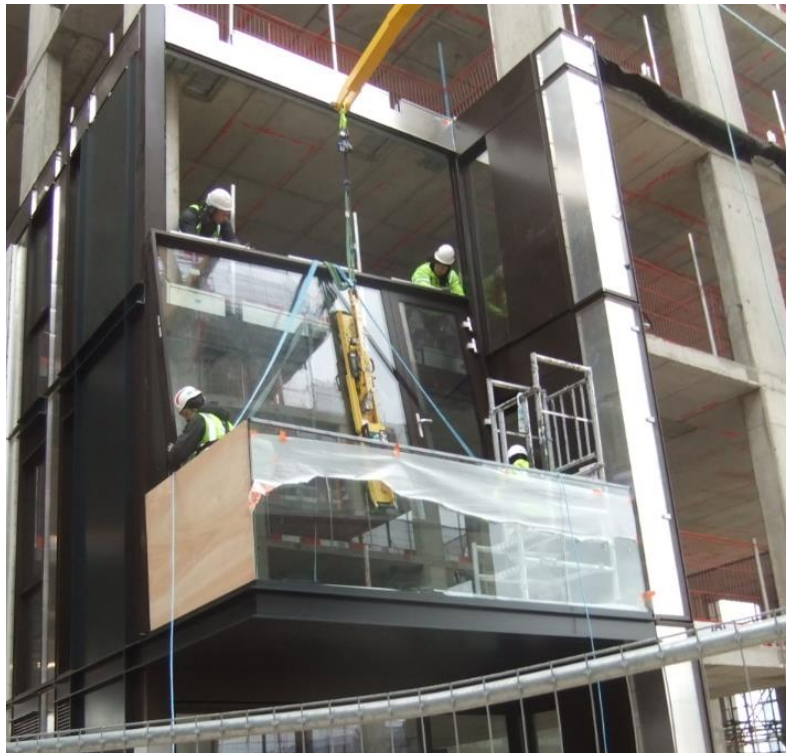
Figure 5.1.12 Building foto's (Scheldebouw, 2019)
