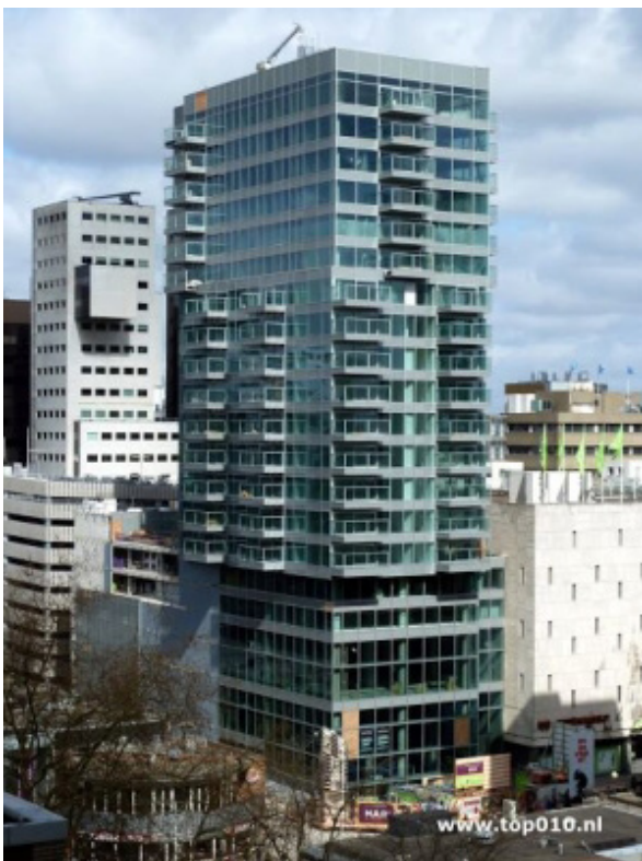
Figure 5.1.09 Building foto's (Scheldebouw, 2019)
