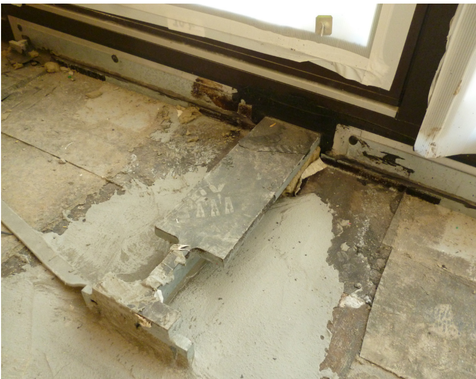
Figure 5.1.13 Building foto's (Scheldebouw, 2019)
