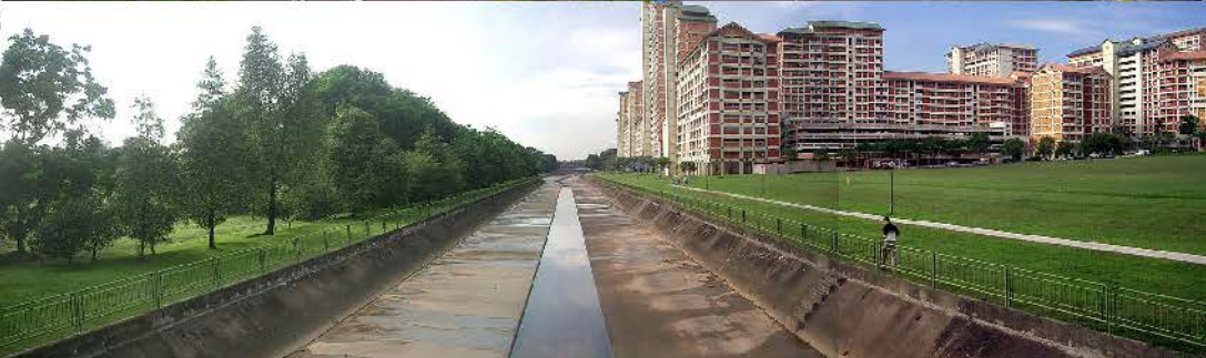
The old Kallang River is an artificial channel to collect and drain the rainwater from nearby urban surface . Photo via wikipedia.
