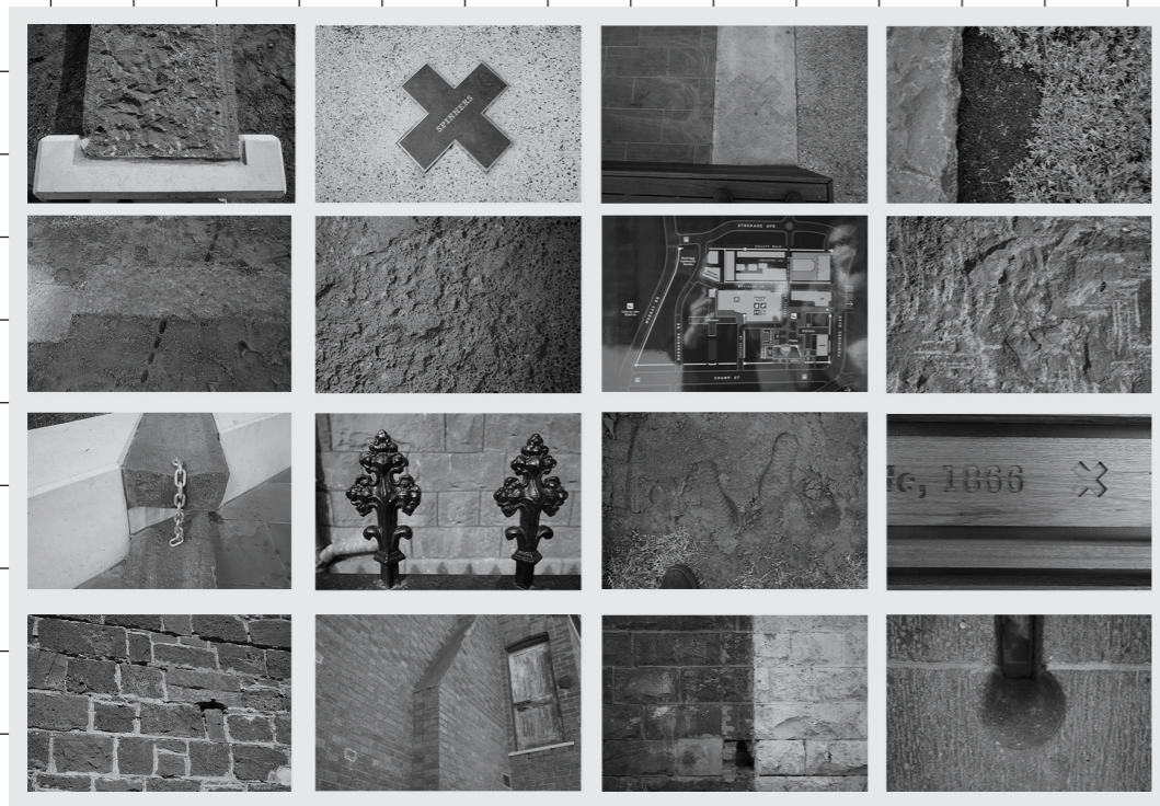
Details of the material textures and arrangements around the Pentridge site. Photographs and compilation by Shanti Sumartojo.
