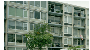
*Figure 1.3.22. 1984 After Renovation: Grid: light brown, Balconies: gray; Parapets were in different colors.
