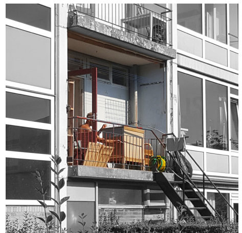
Figure 1.5.48 Balcony for housework
