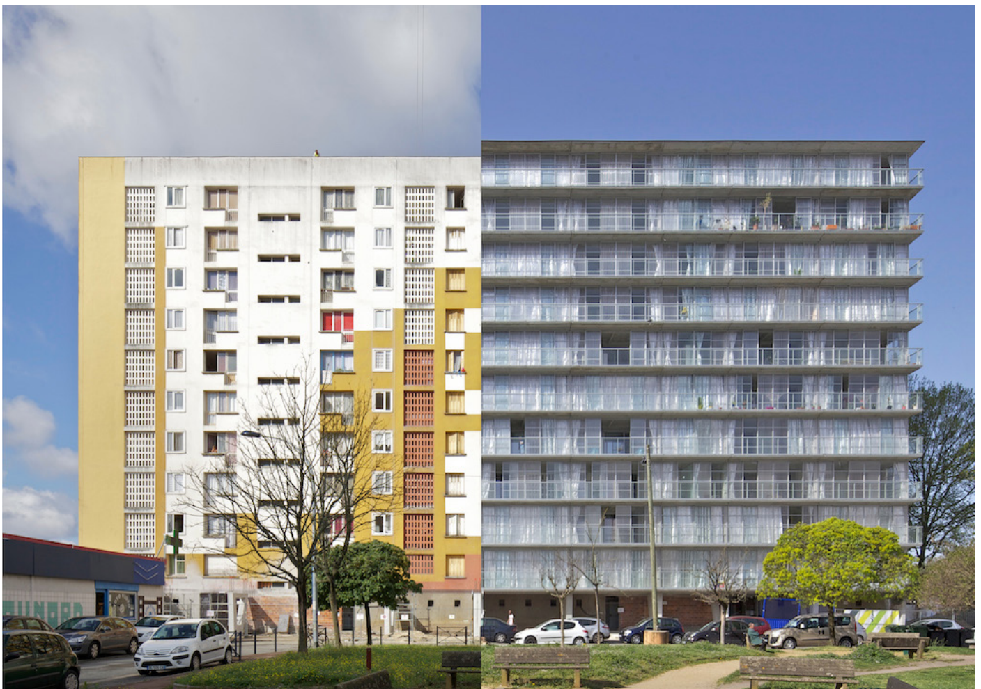
Figure 2.1.2 Elevation of one project renovated in plus approach. Left: original condition; Right: Renovated
