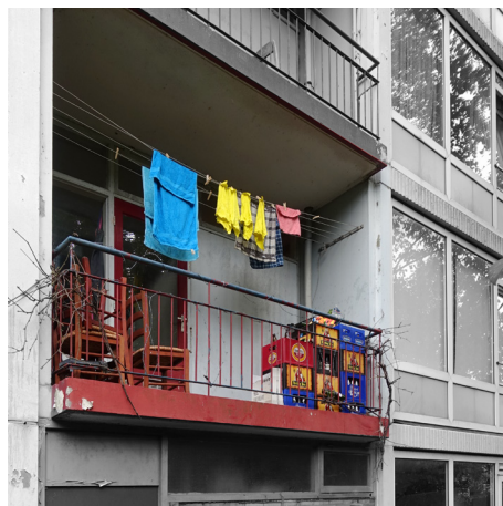
Figure 1.5.47 Balcony for housework
