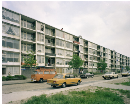
*Figure 1.3.14. 1984: Timber window frame with Single glazing
