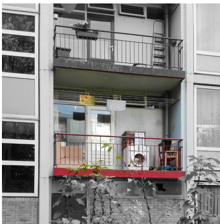
Figure 1.5.46 Balcony for housework
