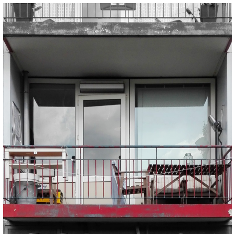
Figure 1.5.52 Balcony for leisure
