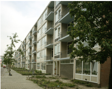
*Figure 1.3.15. 1984 After Renovation: Fall protection was added.
