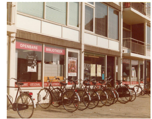
*Figure 1.3.20. 1973-78: Vertical grid painted white; Horizontal grid painted brown; Window frames and parapet white.
