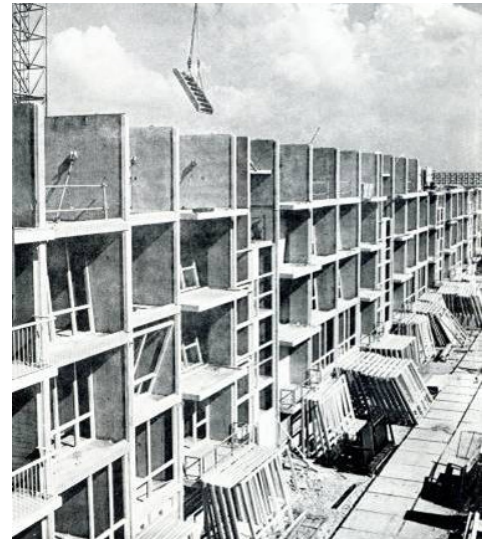
Figure 1.2.3: Assembly on site
