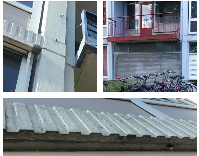
Figure 1.3.5 . Prefabricated fragments attached to structure
