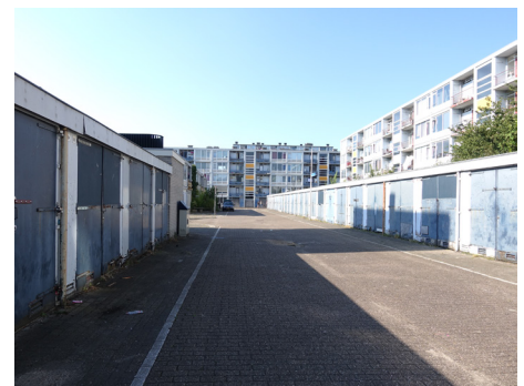
6. The single-storey garages are standing in a row. People can rent the space for 100 euro per month. The area seems disconnected from the surrounding environment.
