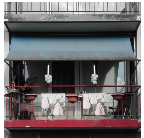
Figure 1.5.53 Balcony for leisure
