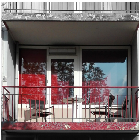
Figure 1.5.51 Balcony for leisure
