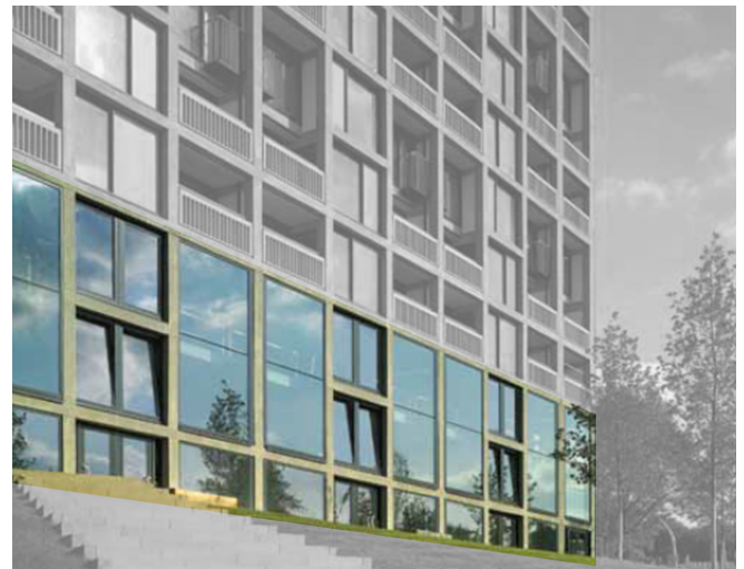
Figure 2.2.13. Ground Floor used as commercial units.
