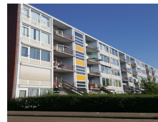
Figure 1.3.23. 2016 Current situation: Balconies and doors: red, Grid: white, Staircases: yellow; Parapets were in different colors.
