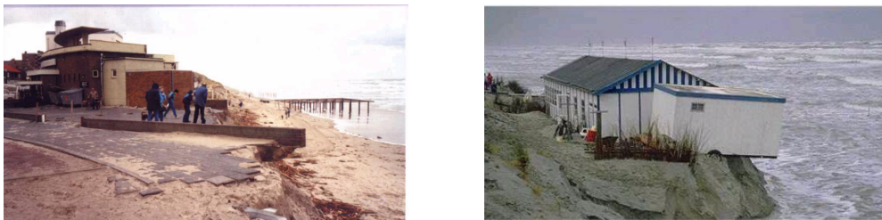
Figure 2.4: Two real examples of a dune erosion on the Dutch coast and the possible consequence of a dune retreat [GoogleEarth].
