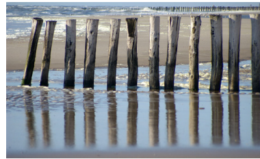
(b) Wooden groyne (area 1).
