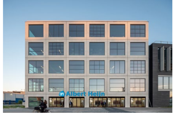
D1. Facade with large storefront (added for survey comparison)
