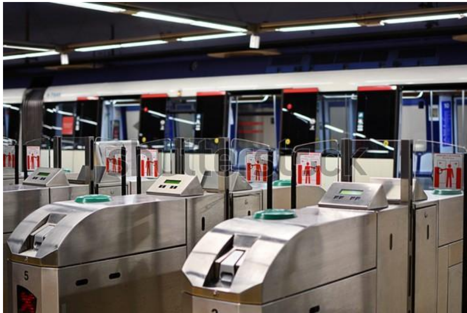
Figure 29: Barcelona subway with customer guidance at front and back of the gate
