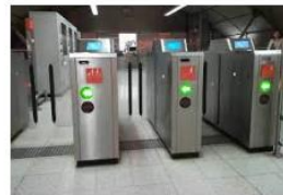
Barcelona subway gates Very quickly retracting Can work 2 ways
