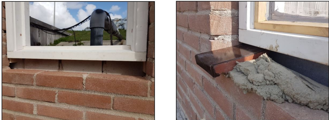
Figure C.7: Placement of the ceramic sills. Underneath the window profile a rebate is present in which the flange of the sill can be locked. Left picture: the situation before placement of the sills. Right picture: sill placement. Note also the small rebate in the sill itself, which is present to allow rainwater to drop in front of the wall instead of seeping over the wall.
