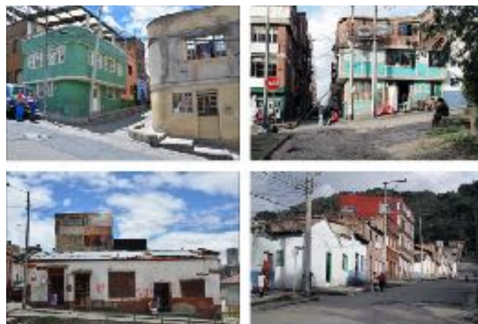
Different building types in la Perseverancia, all of them are largely composed of parts constructed by locals. The proliferation of self-constructions are material manifestation of processes of urban appropriation.
