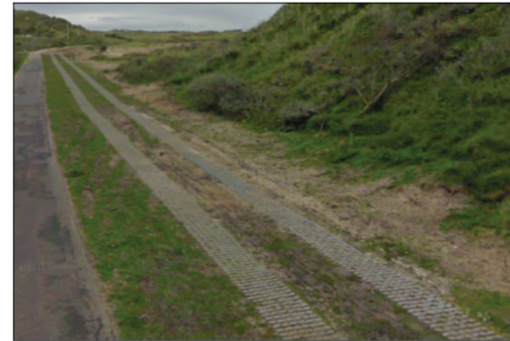
Semi-hardened 3th lane
