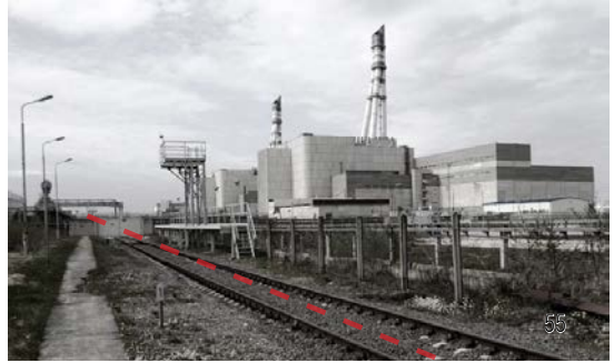
Longitudinal axis is shaped by the buildings on both sides. They create crenelated silhouette. The space is filled with punctual and linear technical elements which cuts the space into smaller subspaces.
