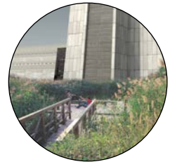
a constructed surface flow wetland (T1)
