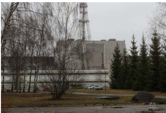
Nature is trying to get into the nuclear power plant site, but is stopped by physical barriers.
