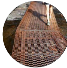
reused steel from demolished INPP buildings
