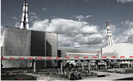
Crossing of two main axis, linear elements and arrangement of reactors defines domination of longitudinal axis.
