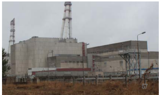
The colors are defined by materials - concrete steel. Technical structures are painted in red or white. Red color is used to highlight important technical structures. Calm color scheme creates the relationships with the surrounding nature. Especially this is visible in autumn.
