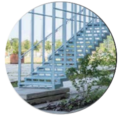
reused steel from demolished INPP buildings
