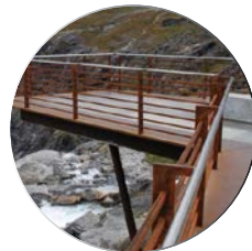
reused steel from demolished INPP buildings
