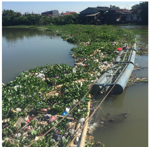
Figure 44: Floating retention boom before Gunung Sari Sluice (Surabaya)
