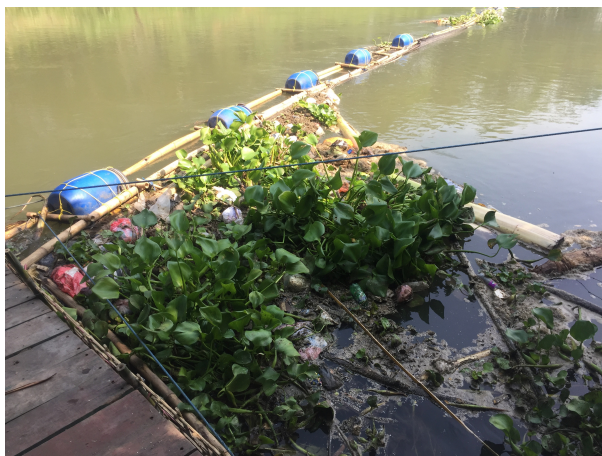
Figure 53: Waste being retained by the floating boom structure
