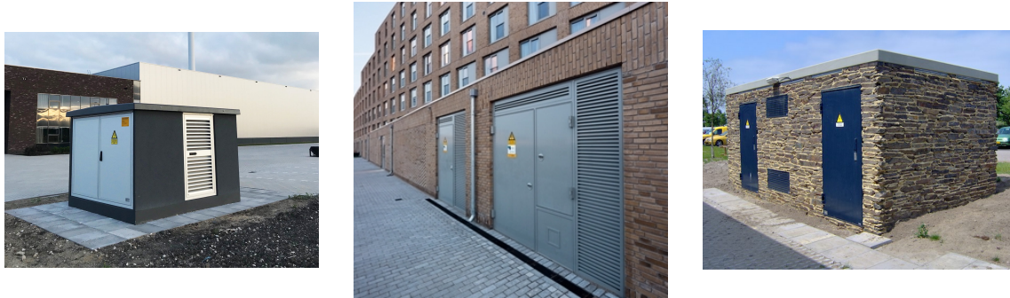
Figure 2.11: Different stations where distribution transformers are in.
