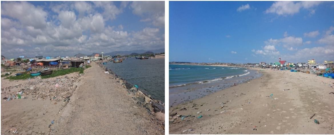
c. A dike near the estuary
