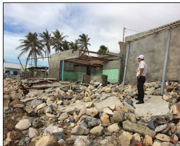
b. Protection after damage and sliding.
