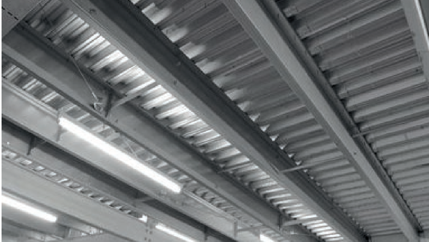
Acoustic roof: perforated steel plates filled with glass or mineral wool
