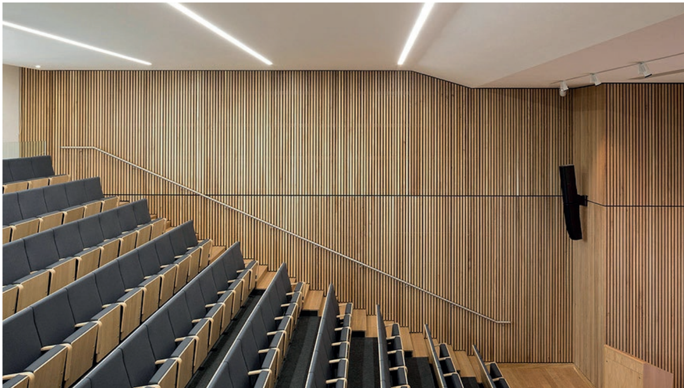
Acoustic walls: slated wooden panels with glasswool behind
