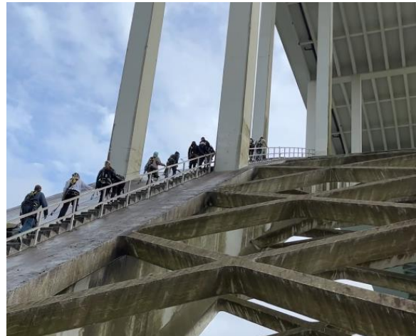
Figure 10: Arrábida Bridge arch climb (Chisholm, 2022)
