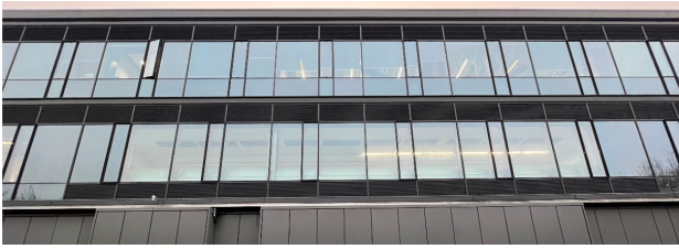
(a) Picture of the building façade
