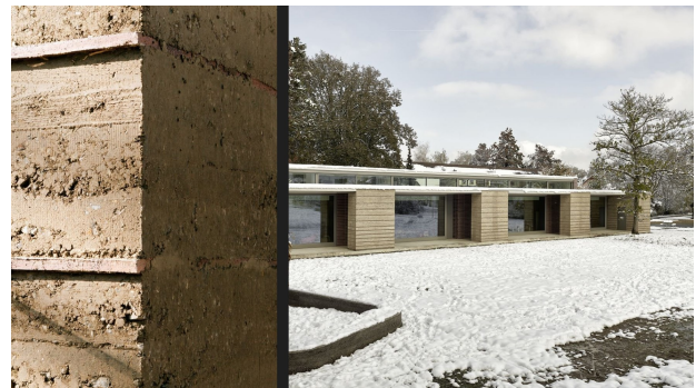
Figure 4: Umbau Schulpavillon Allenmoos II: school with rammed earth walls in Zurich © Boltshauser Architekten
