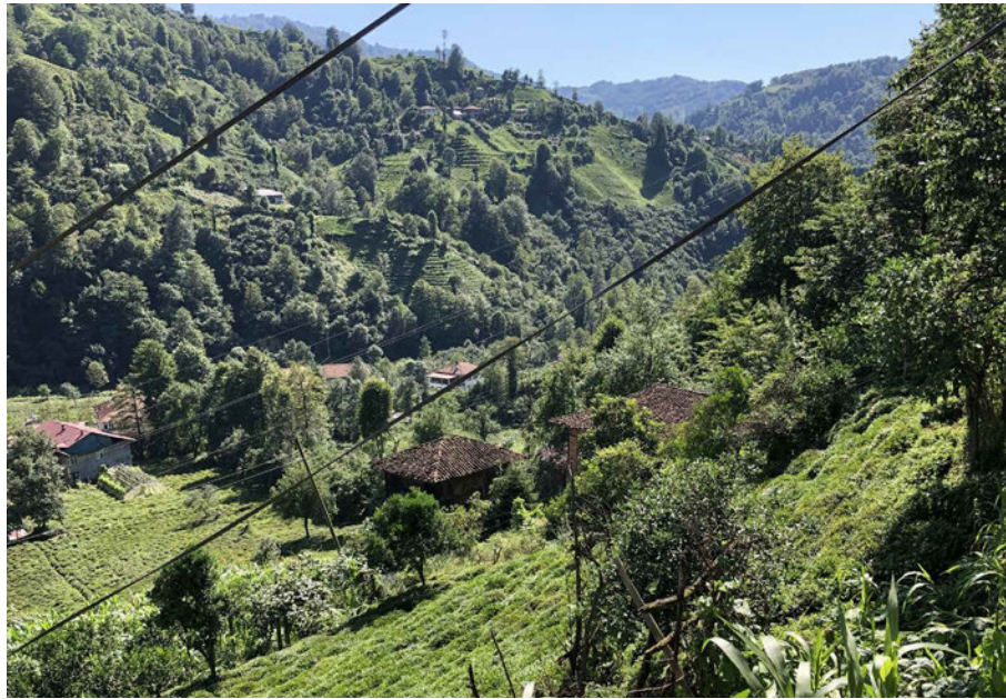
FIG. 3.14 The traditional roof construction of the vernacular buildings is visible at different levels of the steep topography in Arılı village of Fındıklı in Rize. Source: author.
