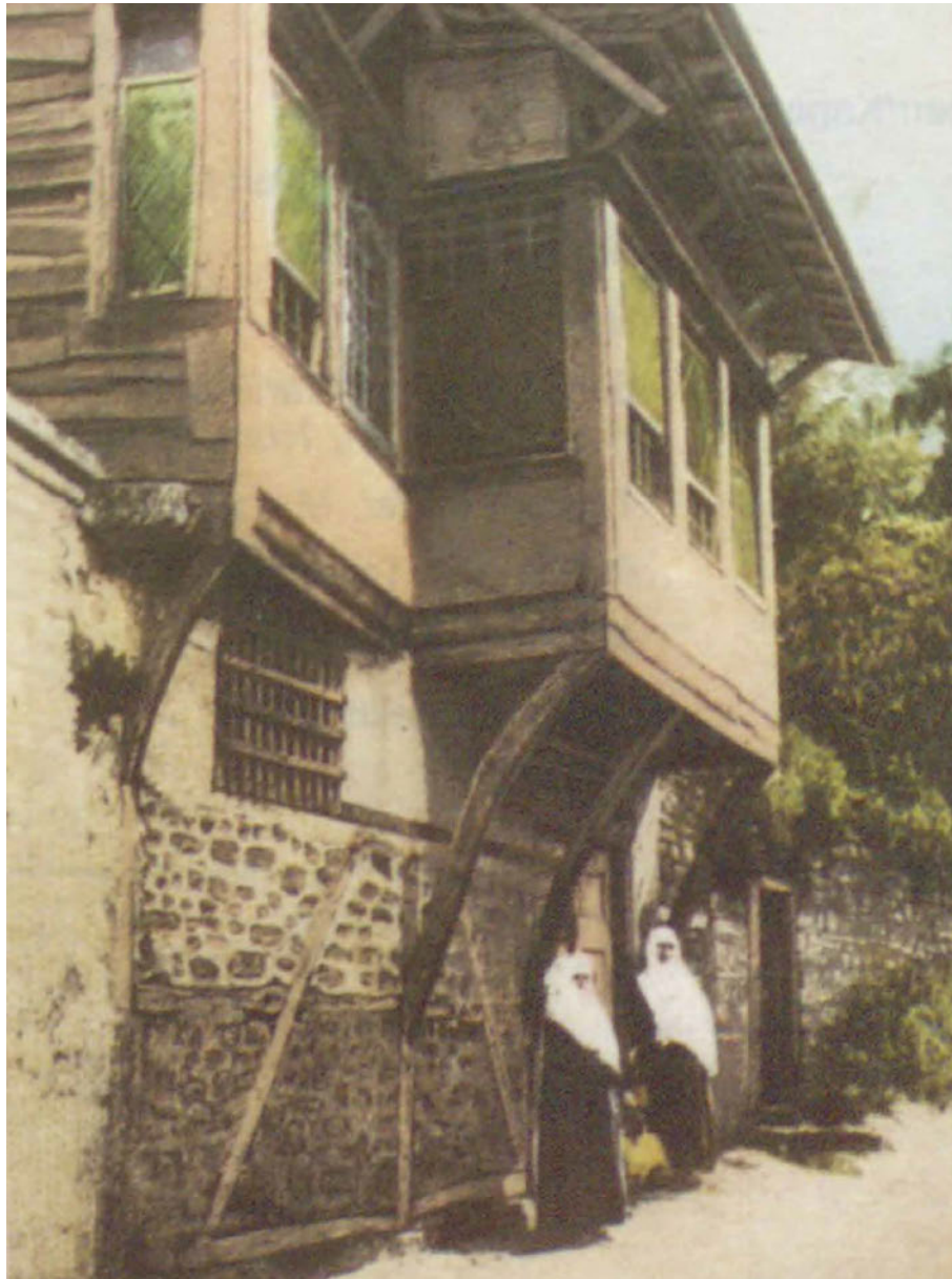
FIG. 2.2 Cumba , 222 also known as a bay window, was used to provide shadow in the streets. Source: Taha Toros Archives.
