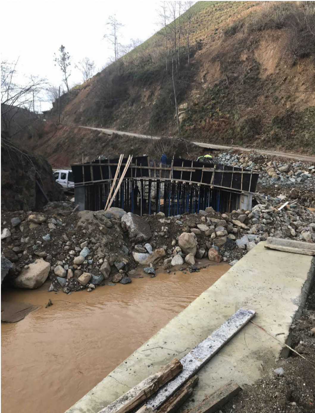
FIG. 5.7 The construction of infrastructure in Çağlayan village and rubble were thrown into the river. Source: author.
