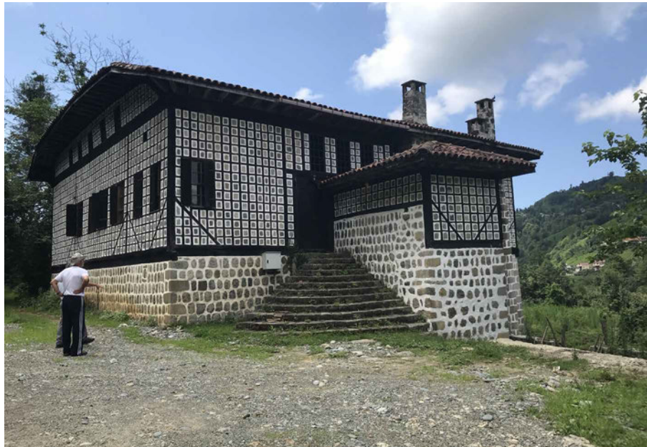
FIG. 4.15 The roof is low pitched and a nice image with its 3-4 ridges. Every room has a fireplace and the stone chimneys connected to these fireplaces extend clear over the peak of the roof. Source: author.
