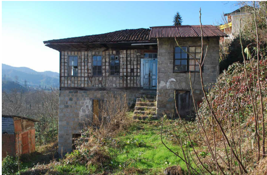
FIG. 4.12 Stone-built façade is facing the steep slope in Çağlayan village. The barn is covering half of the ground floor. Source: author.
