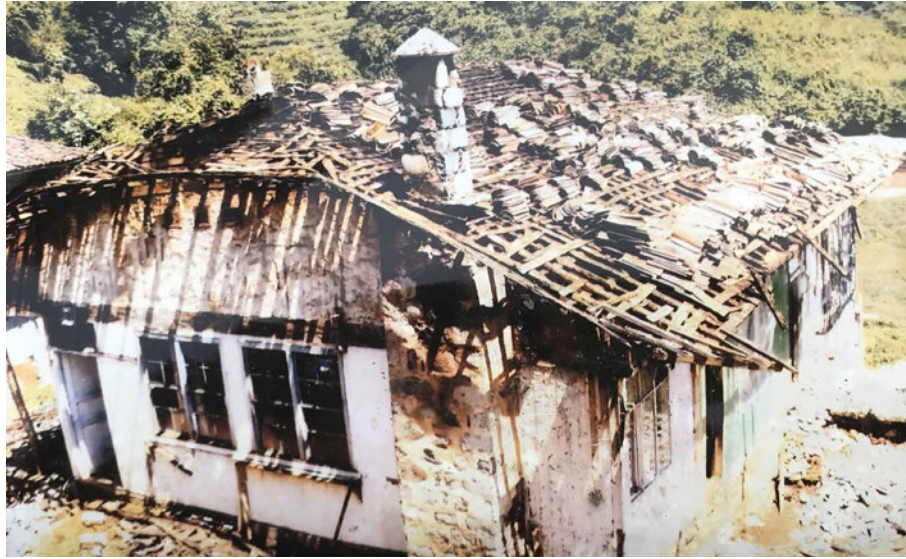
FIG. 6.17 Babalik mansion before and after its renovation shows the skeleton of the timber-framed building. The construction and deconstruction of it always start from the roof, as mentioned in section 3.5. Source: Family archives of the Babalik mansion household.
