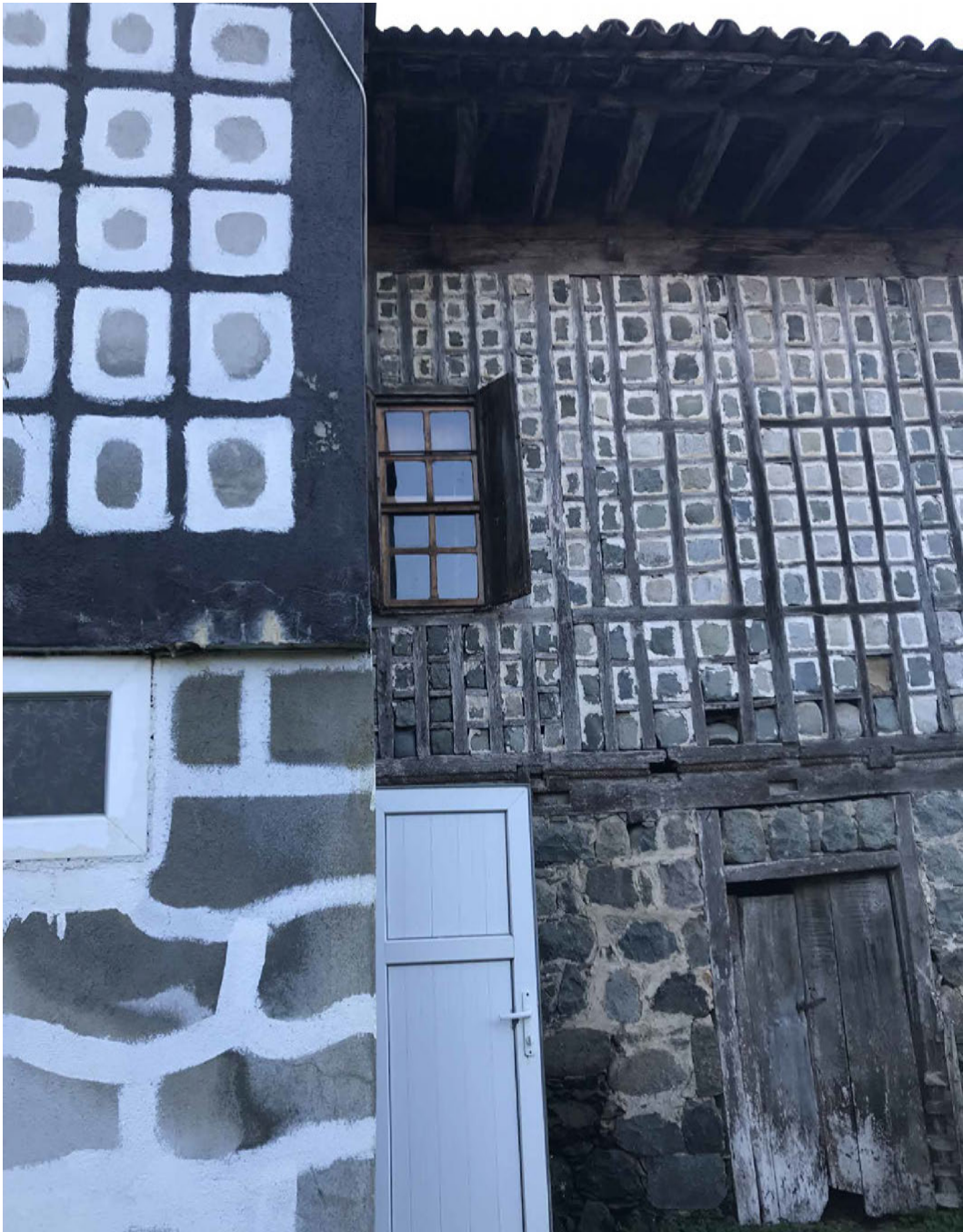
FIG. 6.12 The contrasting view of the original part of the building versus the imitation of stone and stone-infilled timber structure and PVC doors. Source: author.
