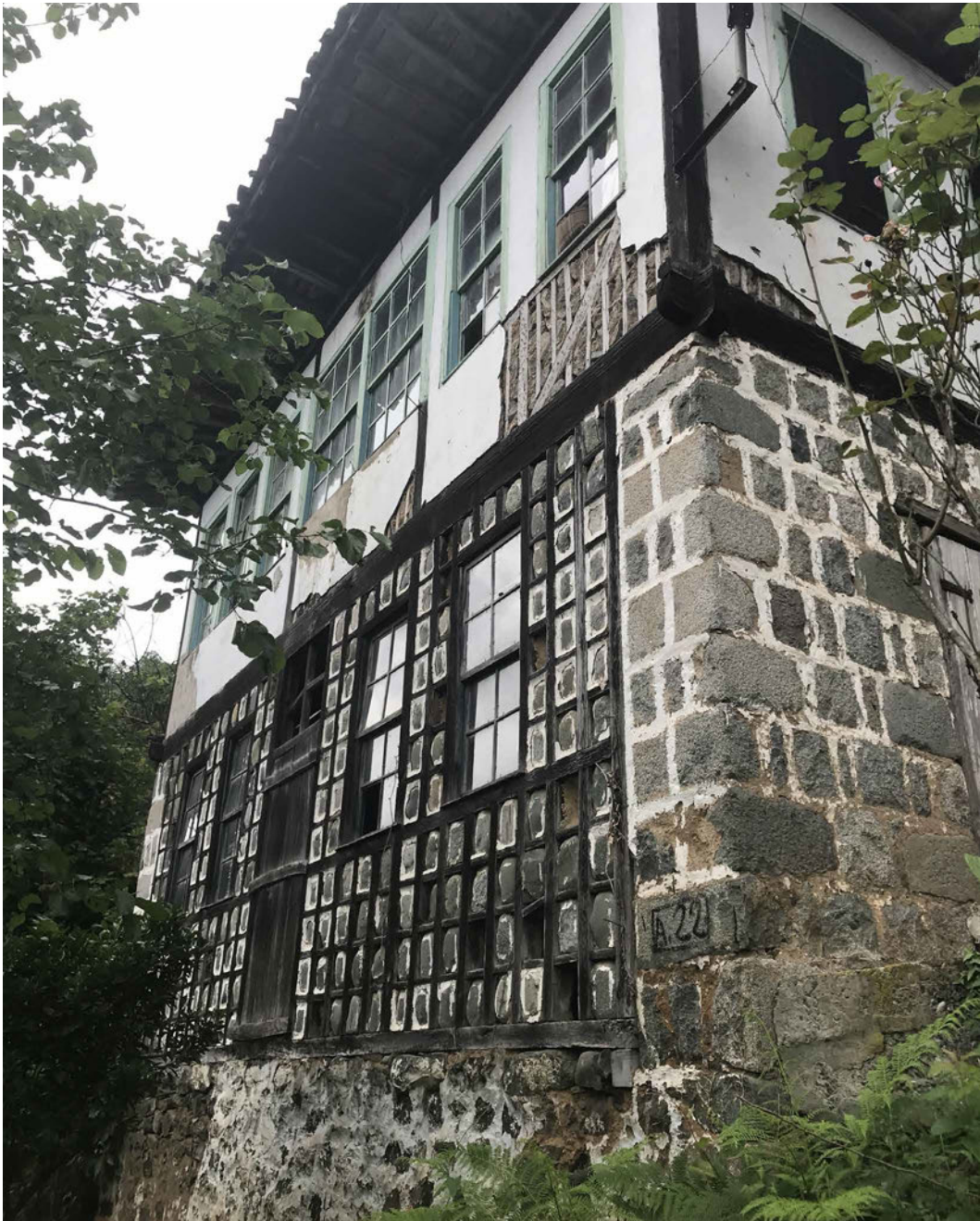
FIG. 3.16 The mixed construction on the façade of O.T. House in Hara village of Fındıklı. The stone and stone-infilled technique on the ground floor and the wooden and plastered façade of the first floor as an example of the cakatura technique. Source: author
