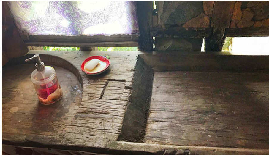
FIG. 4.19 Local people channelled the water through wooden channels to use in washing the laundry and doing the dishes on their timber countertop. Source: author.
