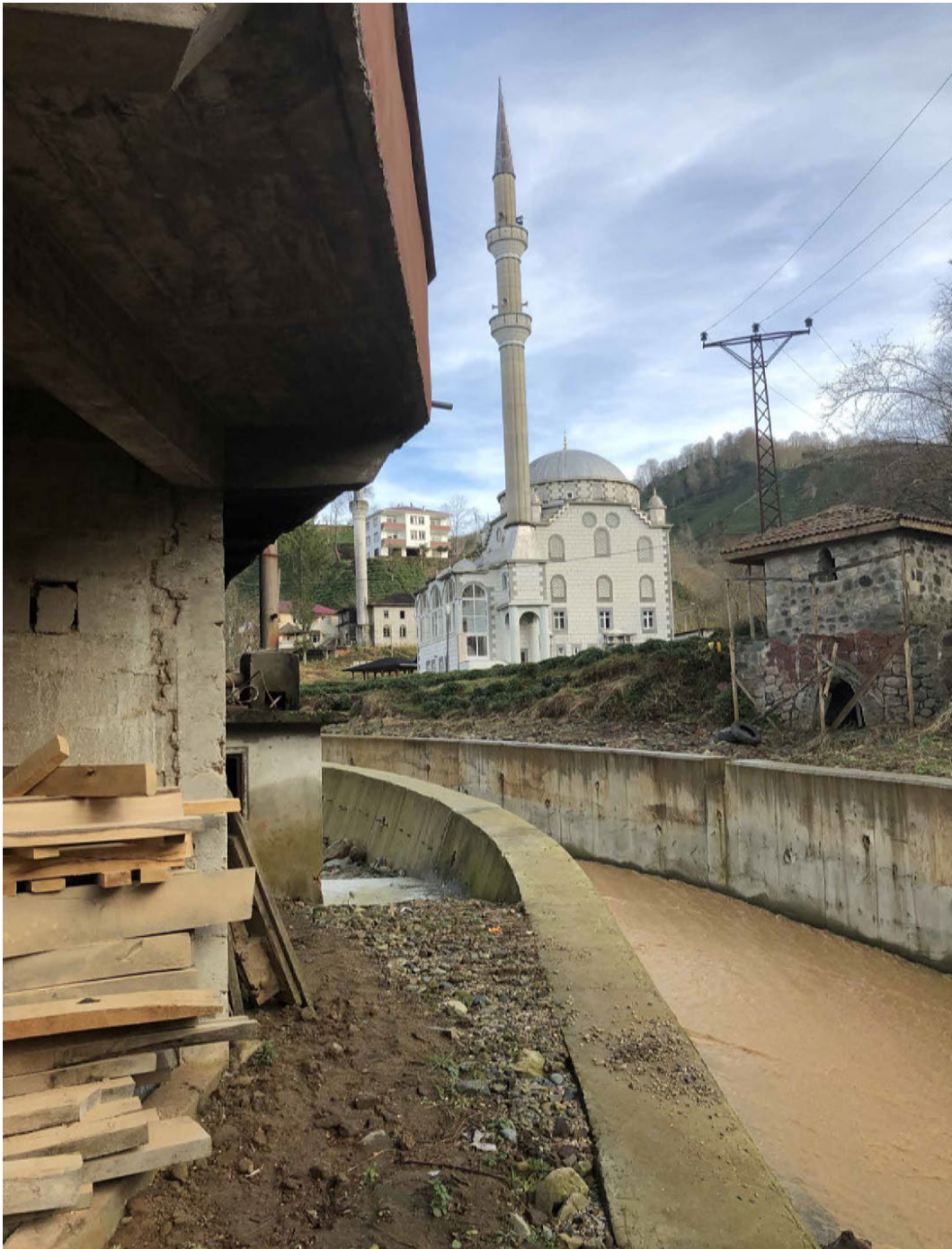
FIG. 5.12 Nearby the river defence wall in Beydere village, there are public buildings such as the mosque. Source: author.
