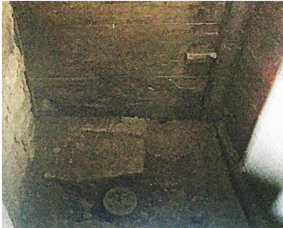
FIG. 4.20 The filter on the floor for water to be drained in the shower in B.T. house in Gürsu village. Source: author.
