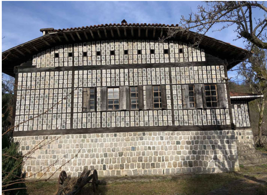
FIG. 4.17 The openings on the rooftop floor allow light inside and airflow inside. A difference in this building is the half floor elevation from the ground to have the barn underneath the building in a lowland area in Çağlayan village. Source: author.
