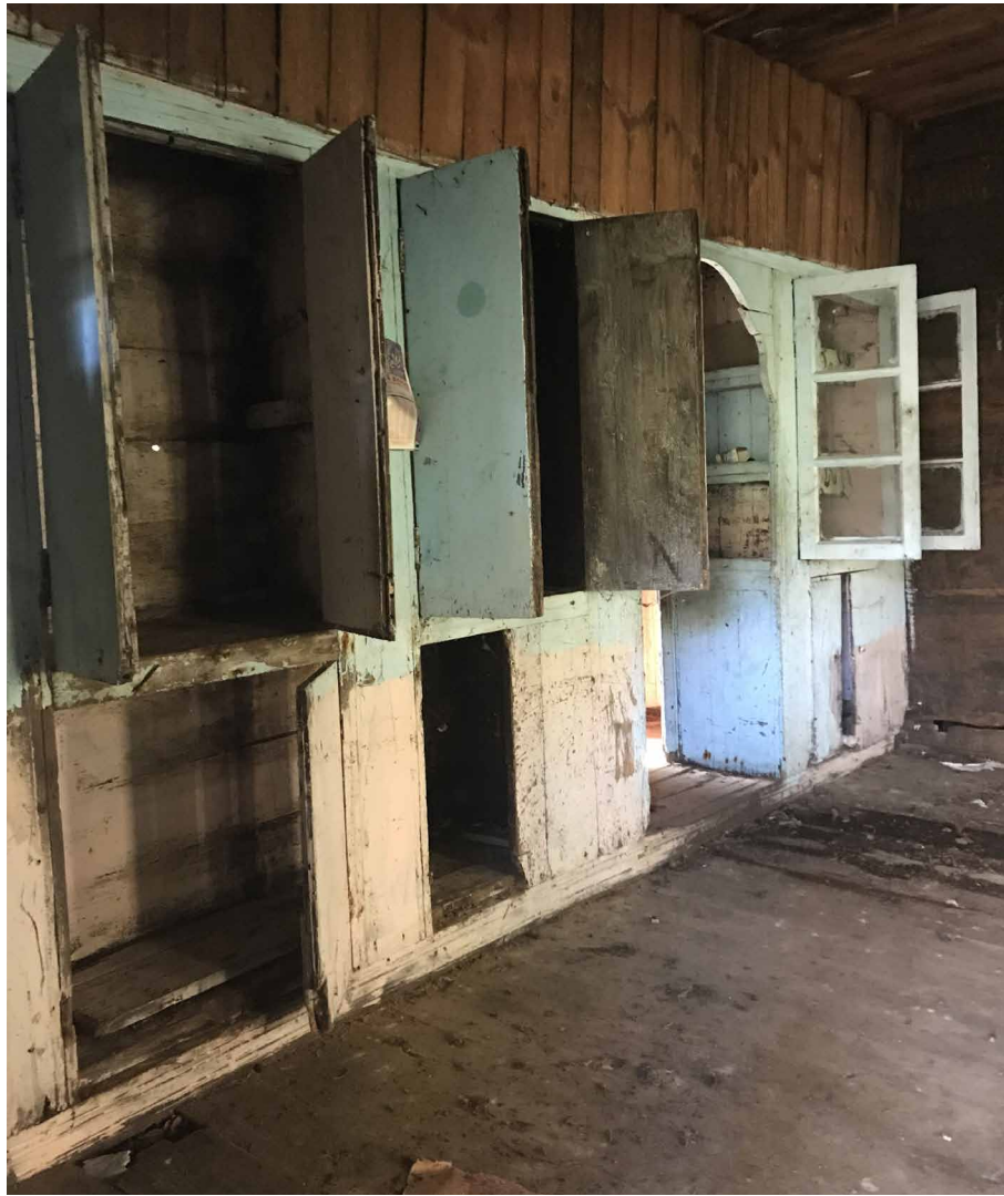
FIG. 4.29 Built-in cupboards in an abandoned building are a humble version of timber cupboards in the area. Source: author.
