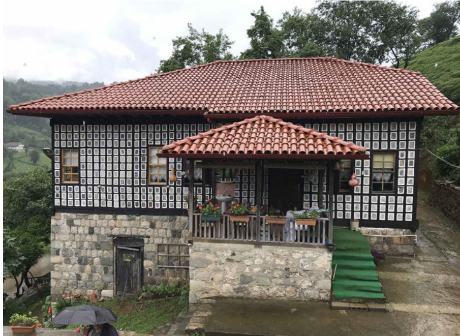
FIG. 6.10 The standalone window on the corner of the façade of the ground floor was accepted as original by the conservation architect. Source: author.
