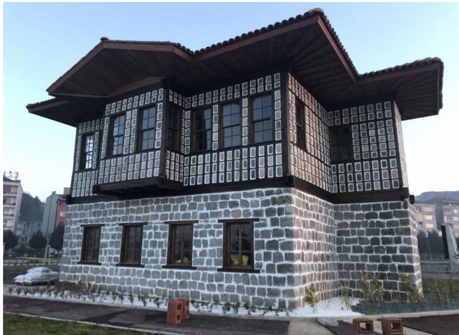
FIG. 6.14 The grand construction of a stone-infilled timber building on the coast by S.S. for the staff of the public institutions to stay during their visit to the district. Source: author.
