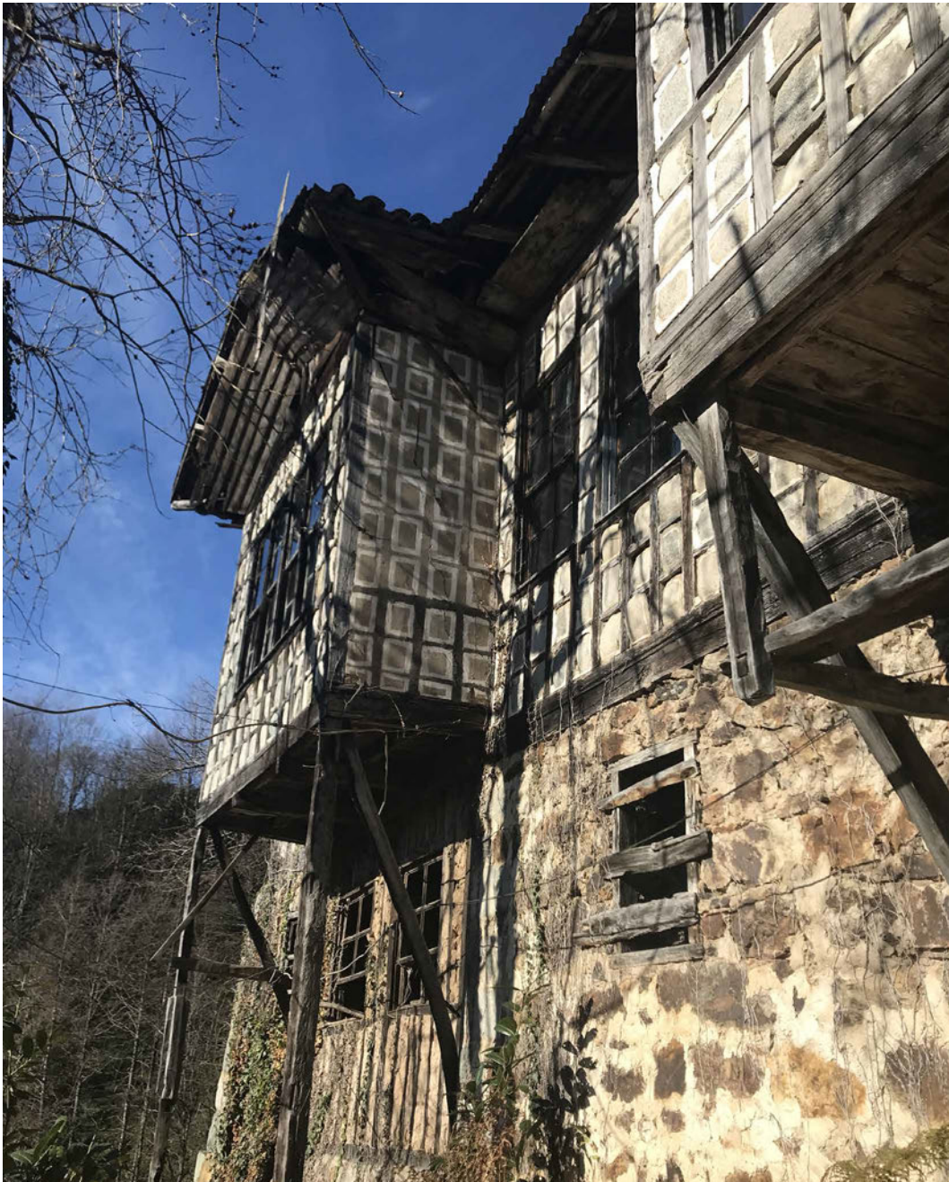
FIG. 4.13 Satiroglu family mansion, which is the only building with two bay windows. These two bay windows create an extra dimension to the living room with a view of the landscape. This is why this building differs from the others in the village of Çağlayan and even in the district of Fındıklı. Source: author.
