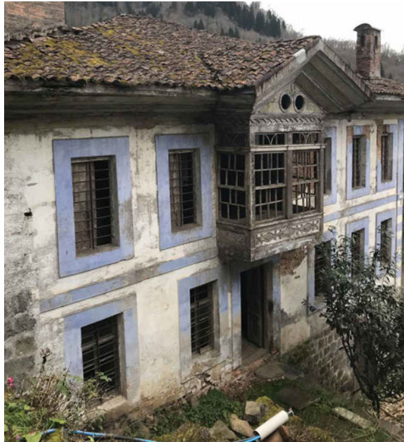
FIG. 3.17 Several interventions from different generations on the building are visible on the facade from wooden, stone-infilled timber, cakatura , stone, and brick materials. Source: author.
