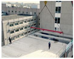
Figure 19 Hollow-core slab floor disassembly and transportation during the demolition process of the Prinsenhof Arnhem (Dycore, 2022)
