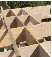
Figure 35 Timber roof structure with dry connections and different lengths. Image retrieved from PLNT (2021)
