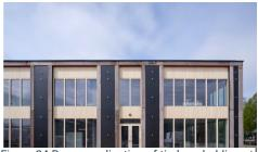
Figure 24 Reuse application of timber cladding at HAVEP project (Paul de Ruiter, 2022)
