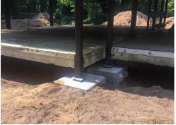
Figure 38 Reused concrete foundation blocks and reused concrete floor slab for a project-specific. Image retrieved from Orga Architecten (2019)
