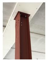
Figure 31 Reused steel column with nuts and bolts which facilitate the disassembly. (Alba Concepts, 2021)
