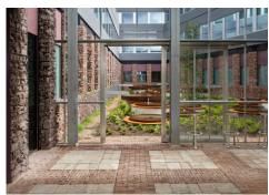
Figure 52 Reused stone tiles and brick flooring at the BioPartner5 project. Image retrieved from Popma ter Steege Architecten (2022)
