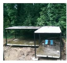
Figure 30 Reused steel with integrated connection from different layers which makes disassembly a challenge. Image retrieved from Cuppens (2019).
