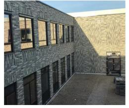
Figure 41 Reused aluminium window frames (Alba Concepts, 2022)
