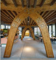
Figure 29 Timber rafter with bolts and nuts connection. Retrieved from SUPERUSE STUDIOS (2020)
