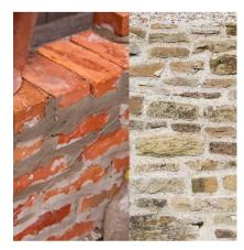
Figure 43 Ceramic cladding with cementbased mortar (left) are more difficult to disassembled without causing irreparable damages. However, when disassembling ceramic cladding with lime-based mortar (right) has a lower damage percentage. Image retrieved from McCoy Mart (2022)
