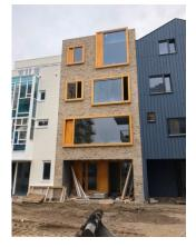
Figure 44 Reused brick cladding and tiles (tiles not visible in the image) (Bouwfonds Property Development, 2020)
