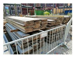
Figure 22 Timber cladding from a renovation project, stored to be later reused in a new built project (Paul de Ruiter Architects, 2021)
