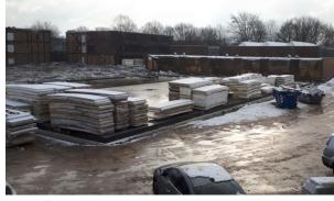
Figure 49 (EPS) insulation used as ground floor insulation is hardly possible to disassemble without causing major damages to the product (Alba Concepts, 2021)
