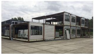
Figure 39 Units to be reused (incl. concrete floor slabs) Image retrieved from Orga Architects (2019)
