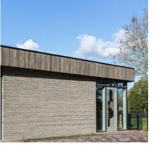
Figure 47 Reused timber roofing profile, scalable aspect of such product is limited to only decreasing its dimensions. (Lucas van der Wee, 2020)
