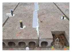
Figure 20 Reuse application of a hollow-core slab floor for the ground floor (Dycore, 2023)
