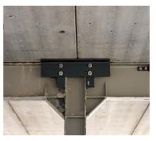
Figure 32 Reused steel construction with added steel connections and bolts which facilitates later the disassembly of this. Image retrieved from Staalprijs (2022)
