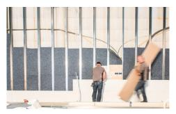
Figure 51 Example of application of reused system walls. Plasterboards are transposed into a horizontal application. Image retrieved from Rijkswaterstaat (n.d.)
