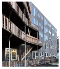
Figure 46 Reused timber cladding at De Warren project. Image retrieved from Natrufied (2023)
