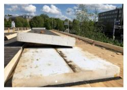
Figure 40 EPS insulation application for new built project. Retrieved from PLNT (2022)
