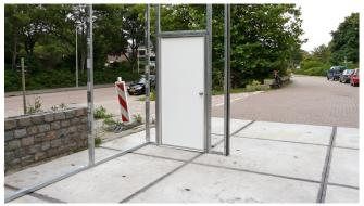
Figure 36 Example of how pre-cast concrete floor slabs can be reused as structure foundation. Image retrieved from Kroftman (n.d.)
