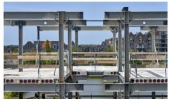
Figure 18 Steel columns for the BioPartner5 project meet the designed height requirements. Image retrieved from Nationale Staalprijs (2023)
