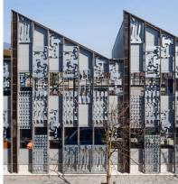
Figure 48 Example of reused aluminium cladding at the waste collection station in The Hague. The disassembly of this type of cladding is easy and does not cause any irreparable damages. Image retrieved from Wessel van Geffen Architecten (2017)
