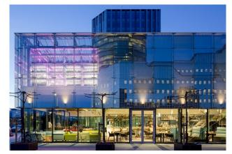
Figure 42 Reused curtain walling at Greenhouse project (Lucas van der Wee, 2018)
