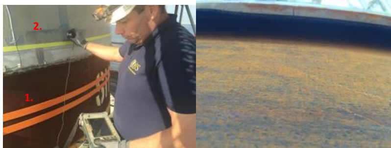
FIGURE 9. WALL THICKNESS MEASUREMENT
