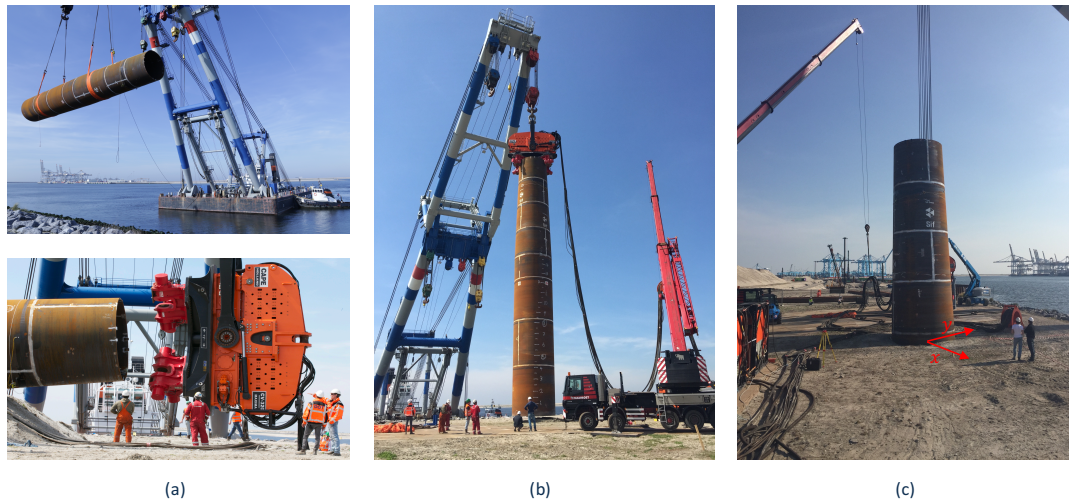
Figure 7.1: Installation phases of day one, the 6th of May
