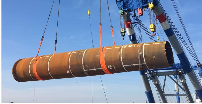
Figure 3.6: Individual plate sections make up the total monopile
