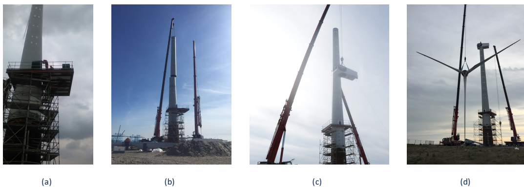
Figure 7.3: Installation phases of day two, the 18th of May
