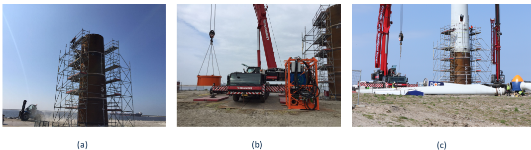
Figure 7.2: Installation phases of day two, the 18th of May
