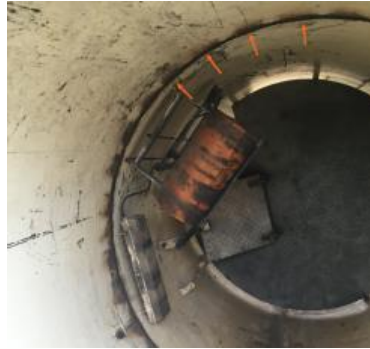
FIGURE 8. WELDS (ORANGE ARROWS) HOLD THE TWO SECTIONS TOGETHER
