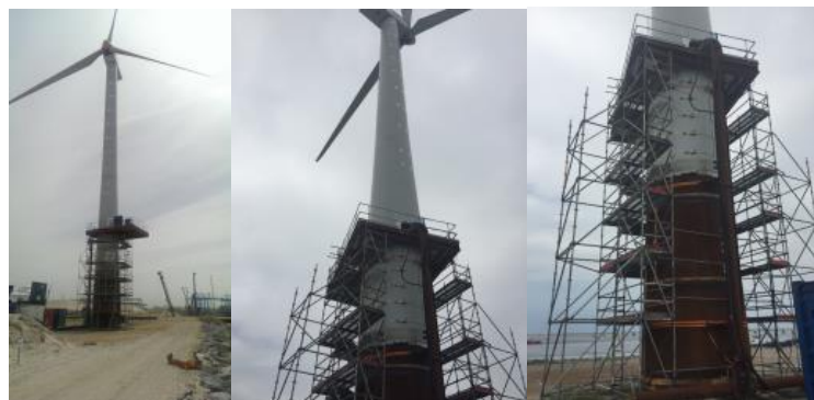
FIGURE 2. DOT SLIP-JOINT AT MAASVLAKTE 2
