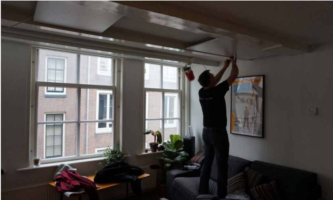
Figure 13: The apartment with Infrared panels on the ceiling [Foto: De Groene Grachten Amsterdam]
