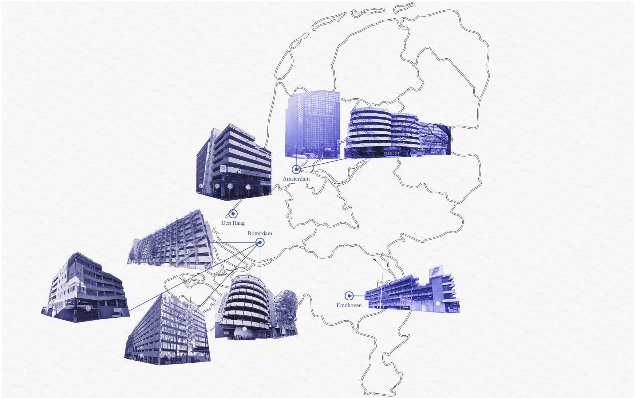
Other multi story parking garages in the Netherlands. Monumental parking garage in a monumental location.
