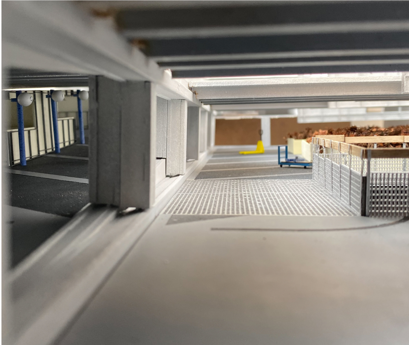
Balustrades made out of reusable metal mesh panels.
