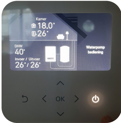
Fig. 10, The incorrect thermostat on the wall intended for professional use
