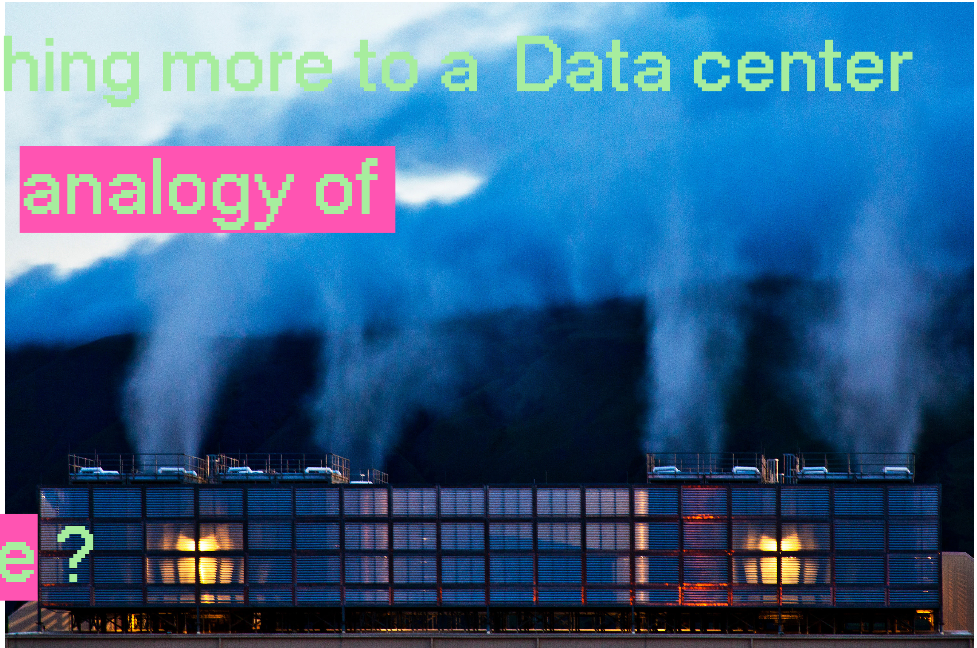
Google Dalles data center in Oregon
