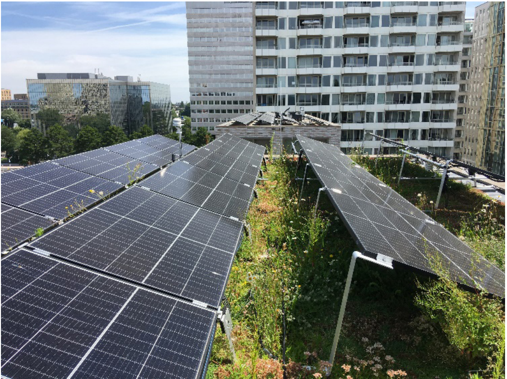
Figure 6.8 Impression of the vegetation in between the PV panels (sunnier area) and under the PV panels (shaded area).
