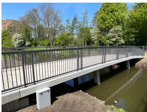
Figure 3.5: Example use of concrete in Pedestrian Bridge (Personal communication, 2024)
