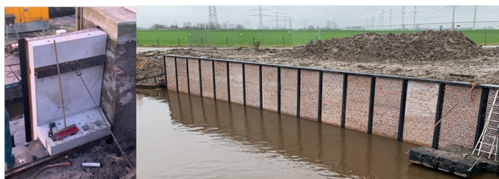
Figure 3.4: Example use of concrete in Quay Wall (Personal communication, 2024)
