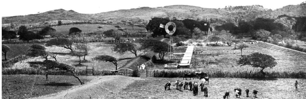
FIG. 15 Windwaterputten (wind-water-well) with series of water reservoirs in the valley of Plantation Savonet around 1900. Between the cattle and the water system a rooi is situated. Large earthen dams are built around the premises as water catchment system. In the hof divi divi trees are planted. Photographer: Soubllette et Fils. Source: RCE.
