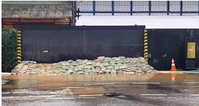
Figure 6 : Reactive flood measure in Porto Alegre, Brazil
