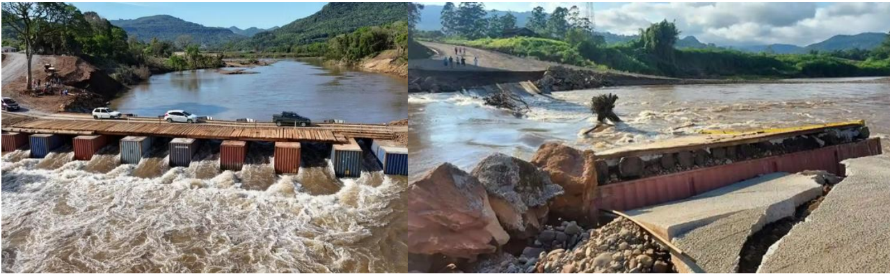
Figure 11 : Temporary bridge built after flood is swept away in Rio Grande do Sul
